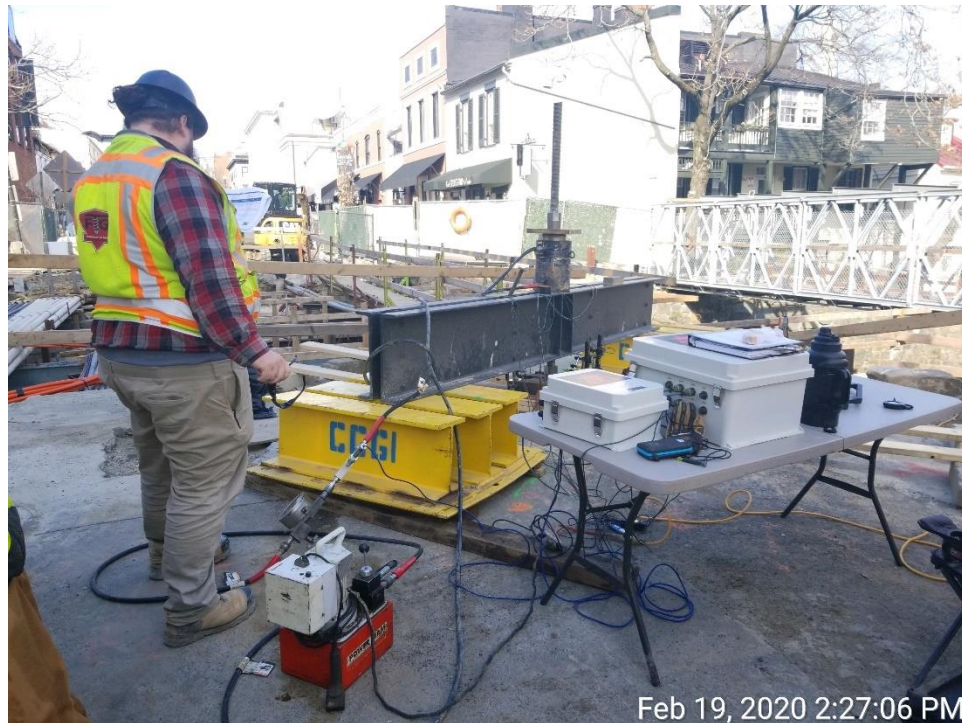
Micropile Load Test – South Abutment
