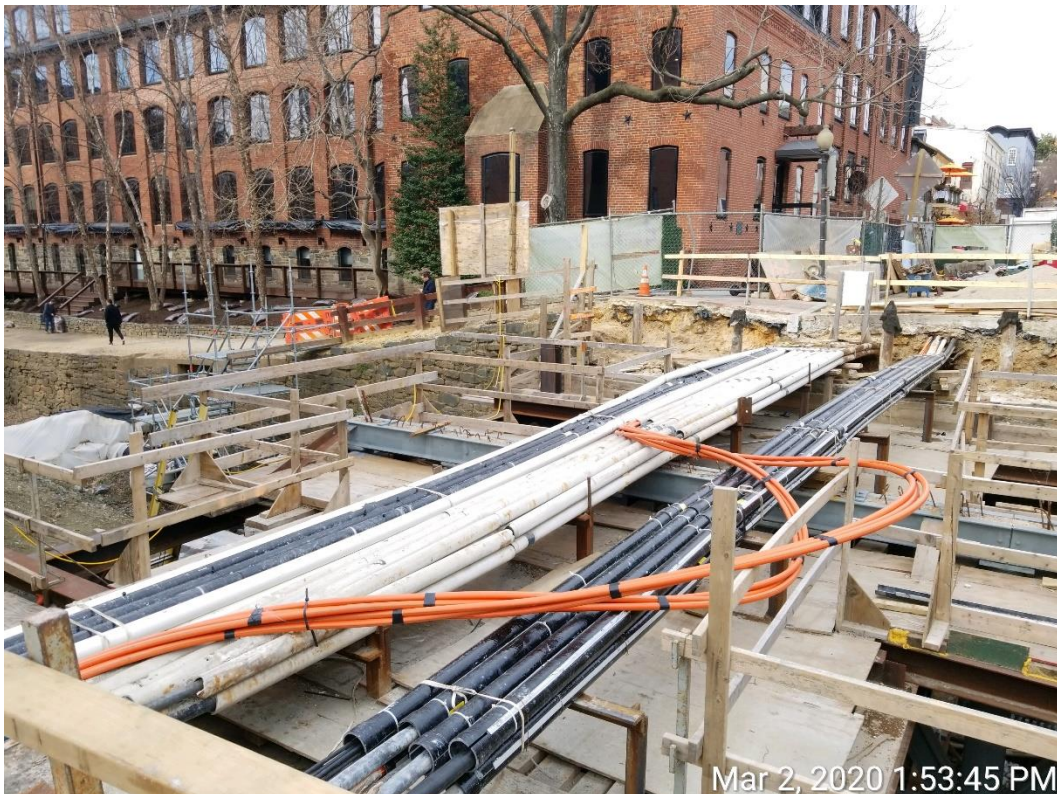
31 ST Street Bridge over C&O Canal
