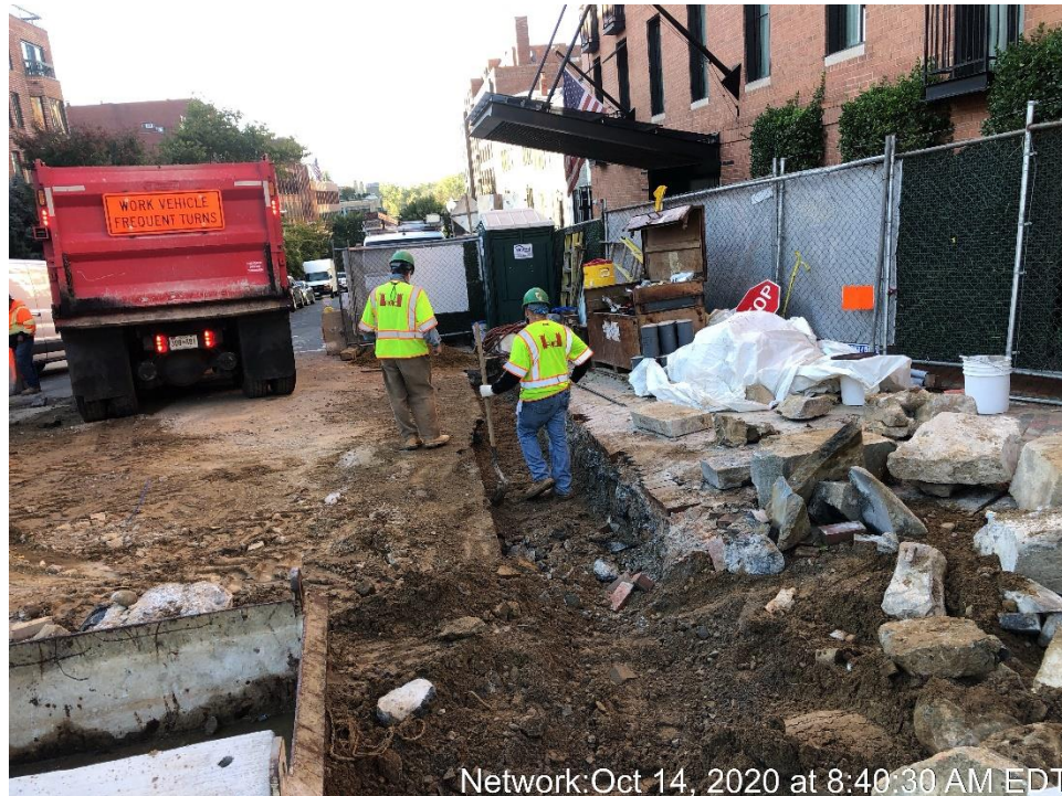
Demolition of the Existing Granite Curb – SW Corner
