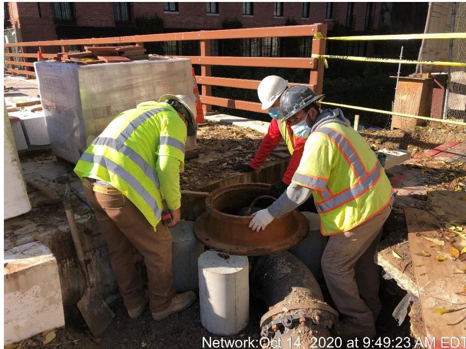
Installation of Blow Off Valve for the 12-Inch Water line
