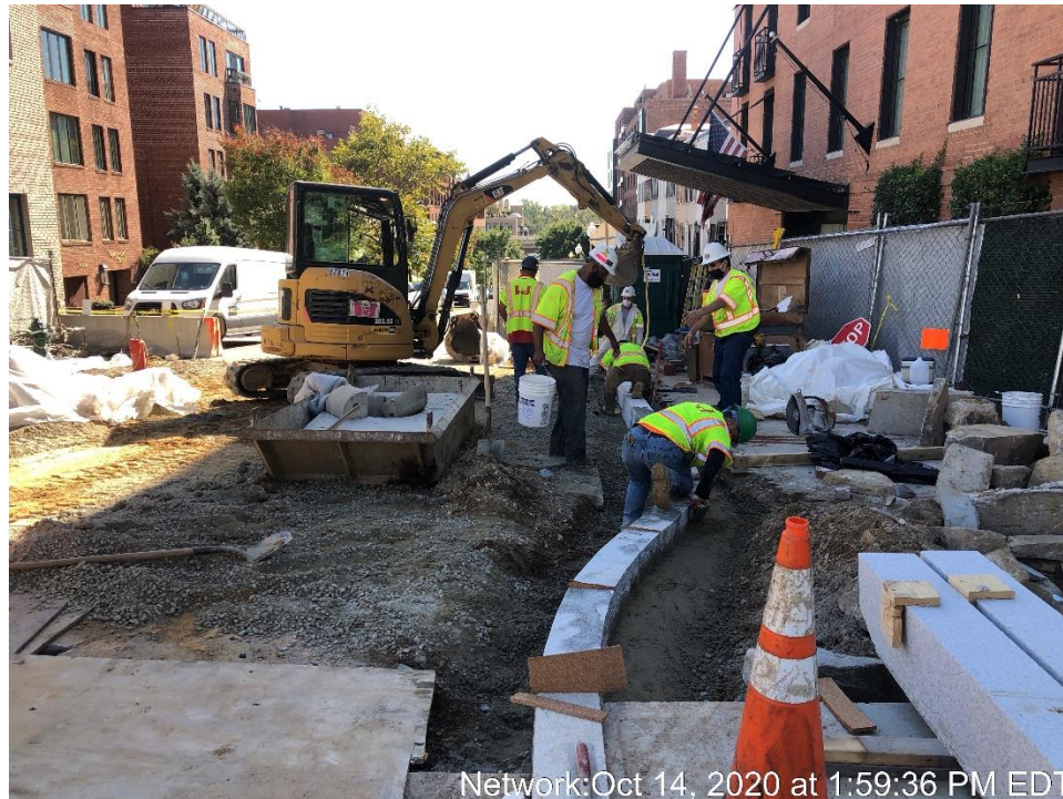
Installation of Granite Curb at SW Side of the Bridge
