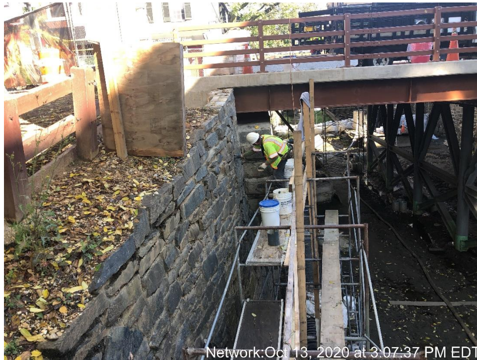
Repairing and Repointing at the North Canal Wall
