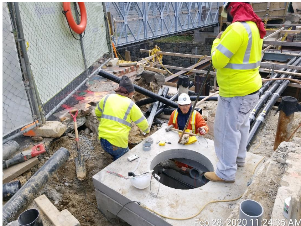
Pepco Work – Connecting the New Conduits to the New MH
