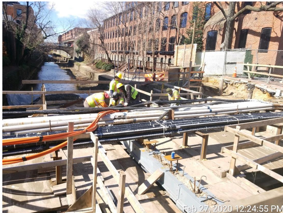
Relocation of Verizon Cables (by others)
