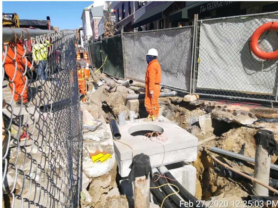
Pepco Work – Installation of new 4-foot x 4-foot Manhole
