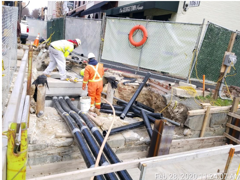
Pepco work – Connecting the New Conduits to the New Manhole
