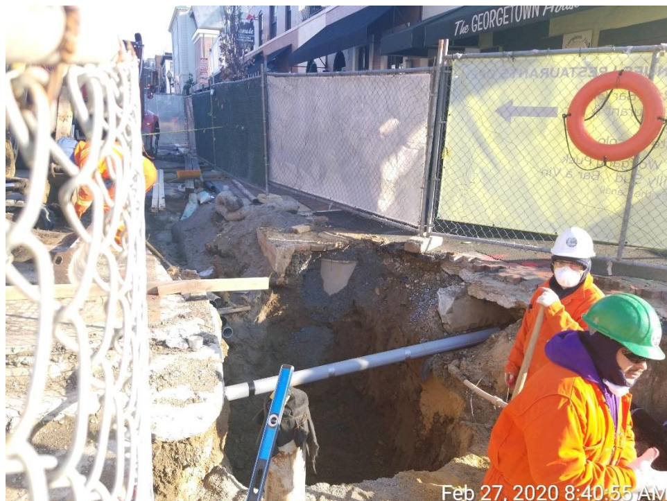
Pepco Work – Excavation for the New Manhole
