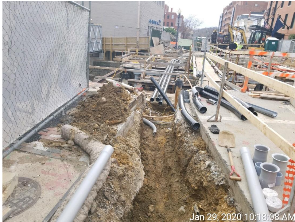
North Side of the Bridge – Pepco Relocation
