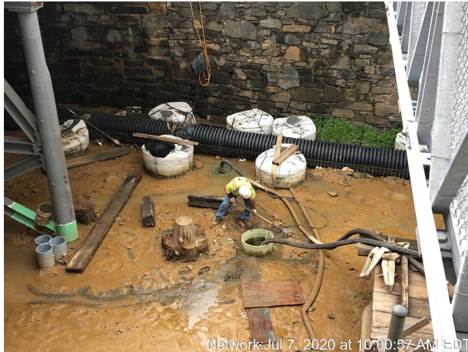
De-watering Flooded Work Zone
