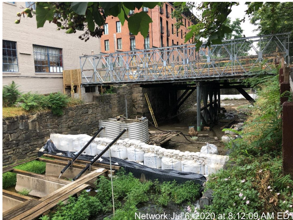
De-watering Flooded Work Zone
