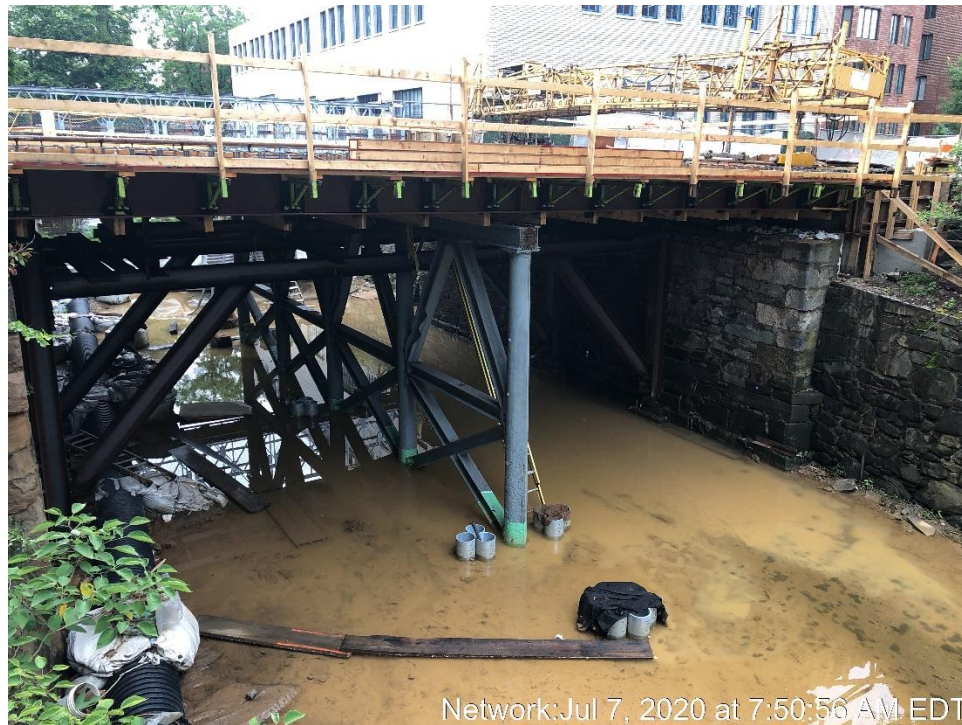
De-watering Flooded Work Zone
