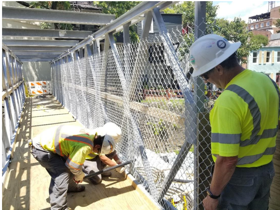
Installation of Steel Chain Link Fence on the Pedestrian Bridge
