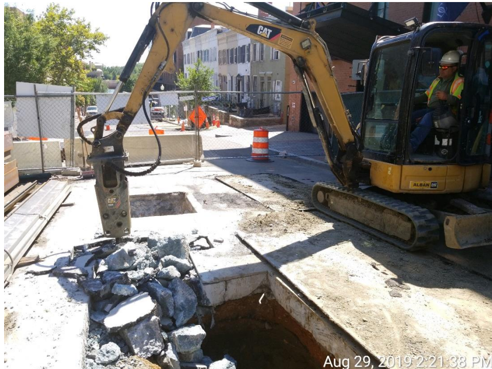
Excavation for the Water Main Relocation at the South Side of the Bridge
