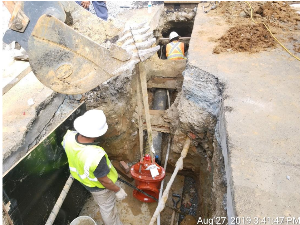
Installation of 8-Inch DIP Butterfly Valve
