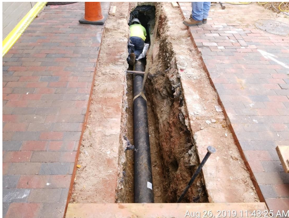
Installation of 8-Inch DIP Water Main
