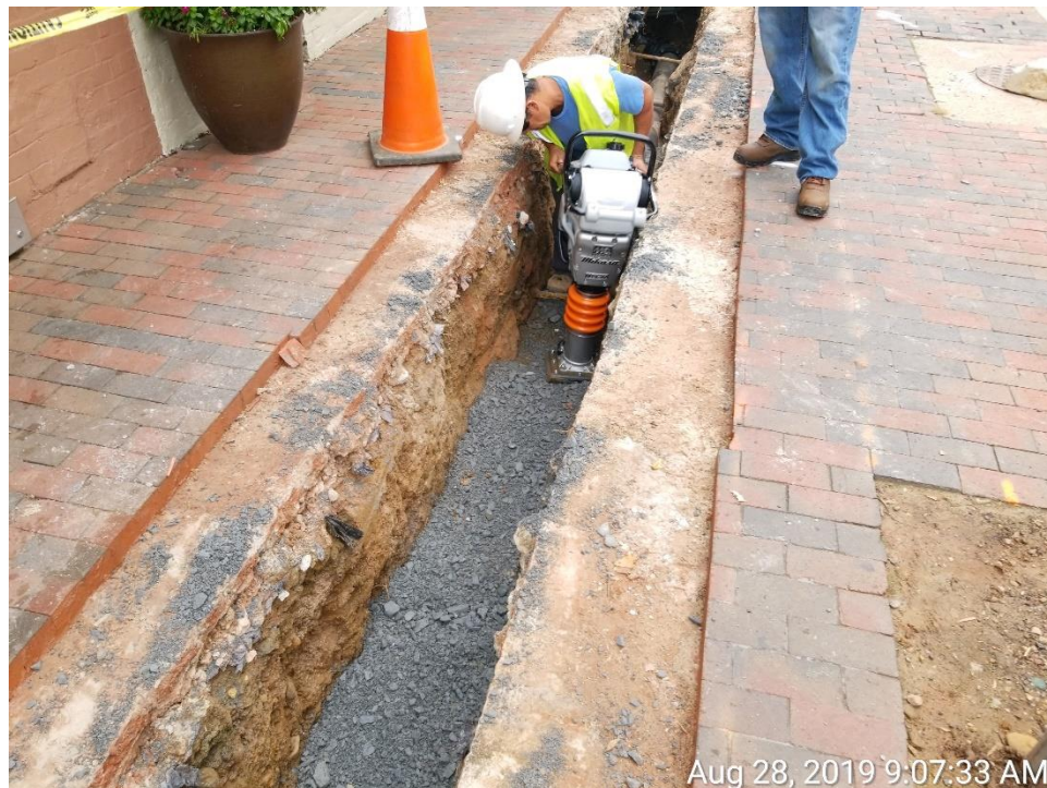
Backfilling the 8-Inch Water Main Trench
