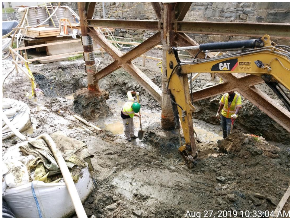
Pier Footings Excavation
