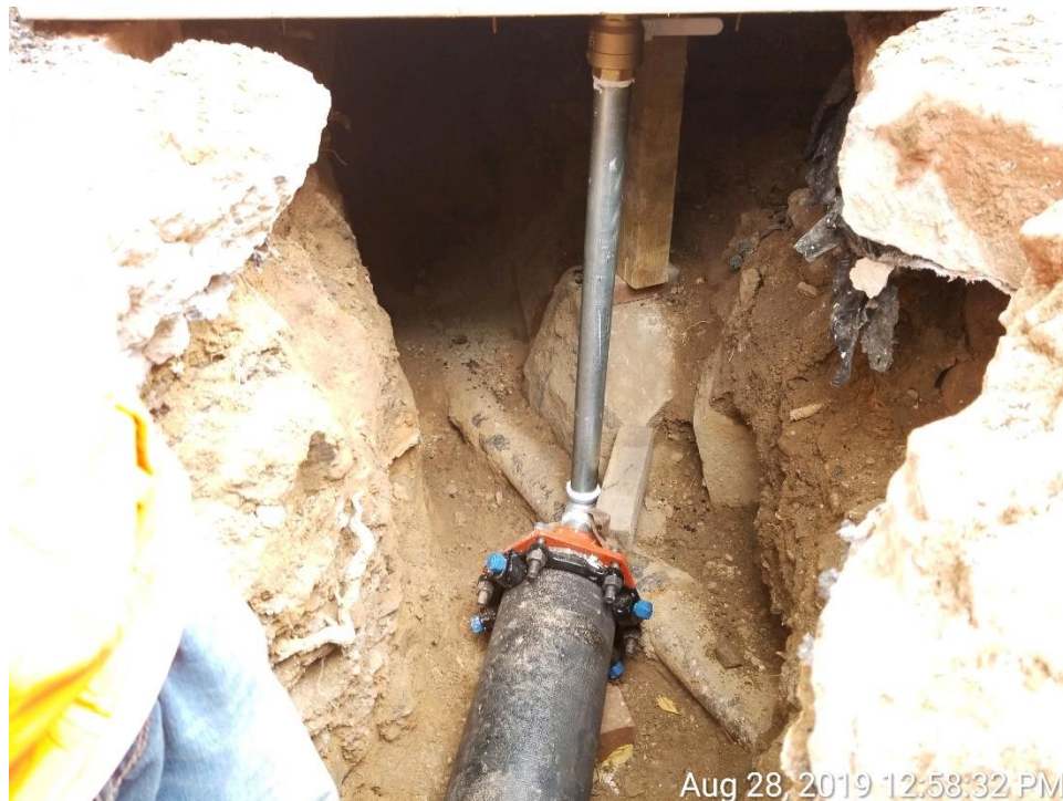
Installation of Water Main End Section at the North Side of the Bridge
