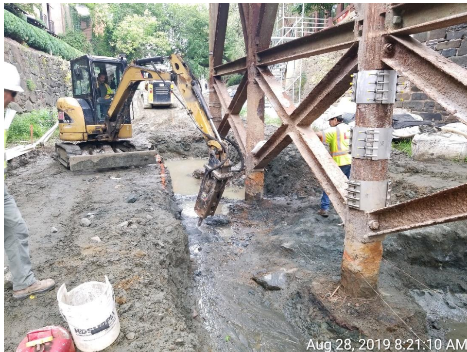
Pier Footings - Rock Excavation at Columns #3 &amp; #4
