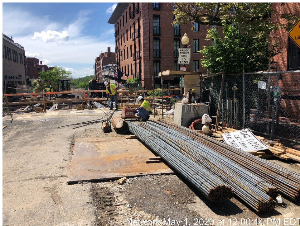
Pier Footing Rebar Work – Bending
