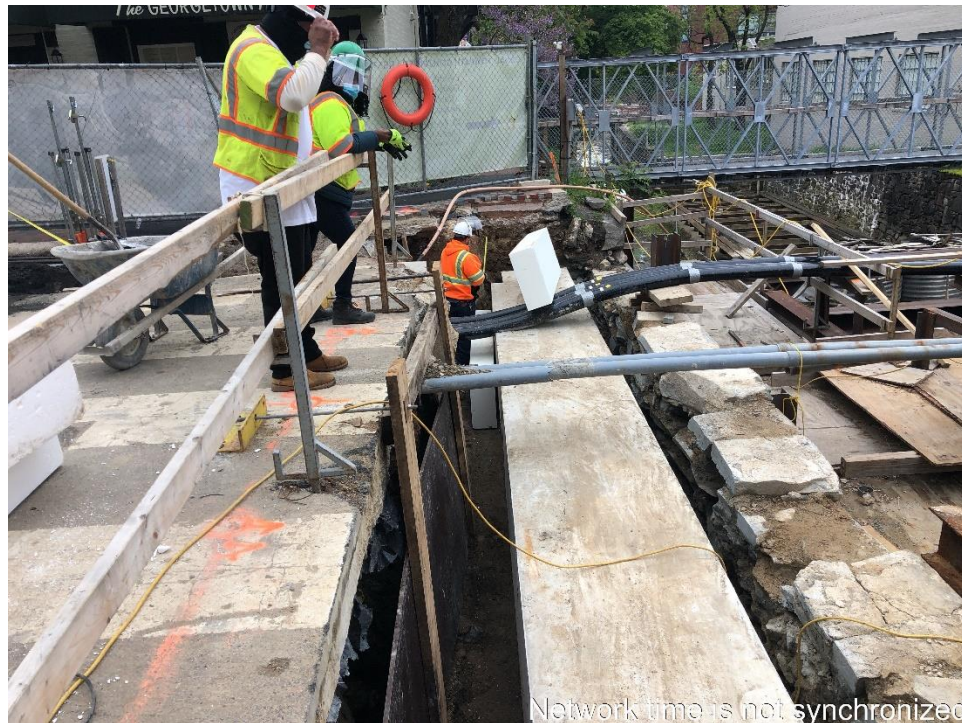
Installation of 10-inch EPS Around the North Abutment Foundation
