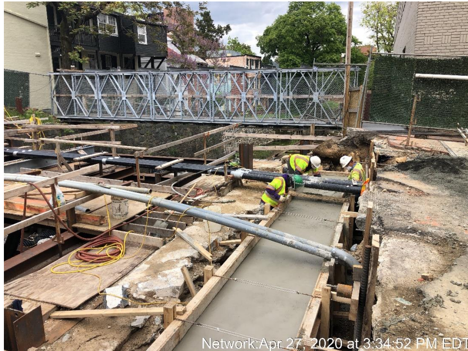
Placement of Concrete for the South Abutment Foundation
