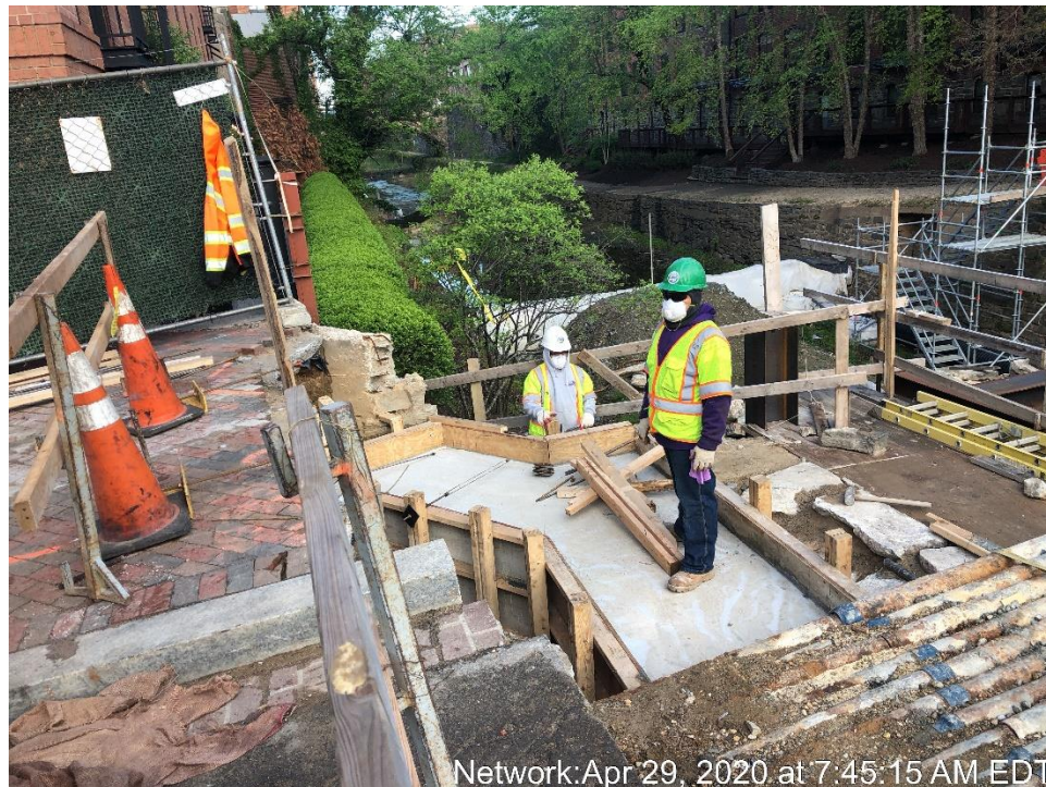
Removal of Formwork at the South Abutment Foundation
