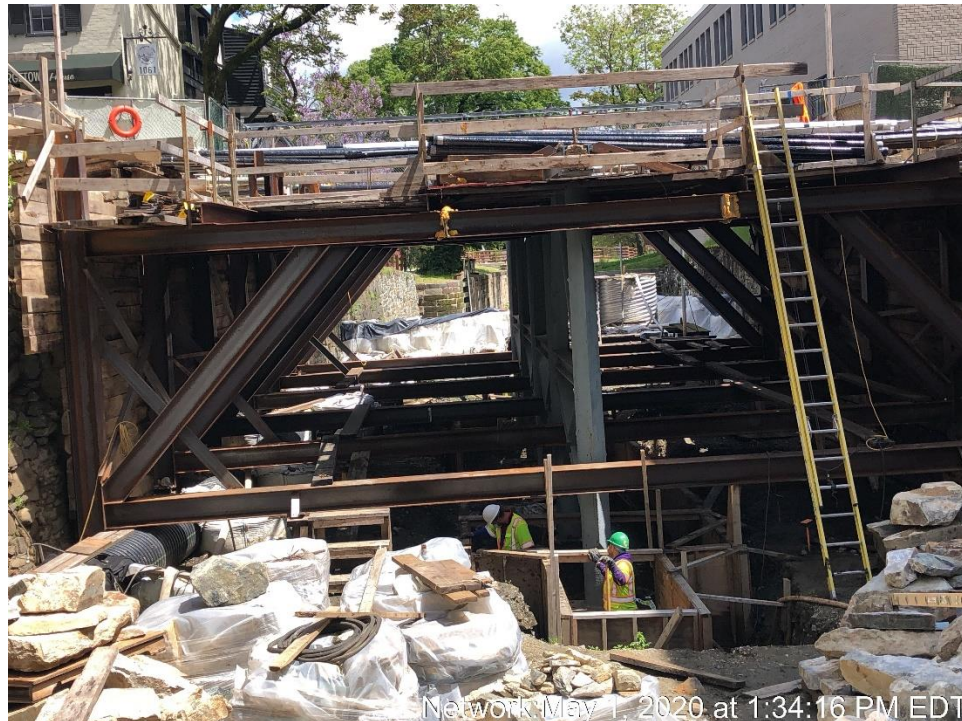
Cleaning the Pier Footing Formwork
