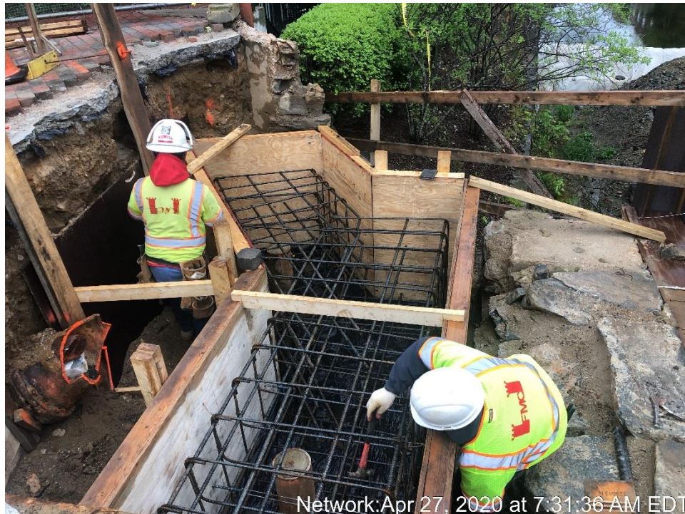
Placement of Reinforcing Steel at the South Abutment Foundation
