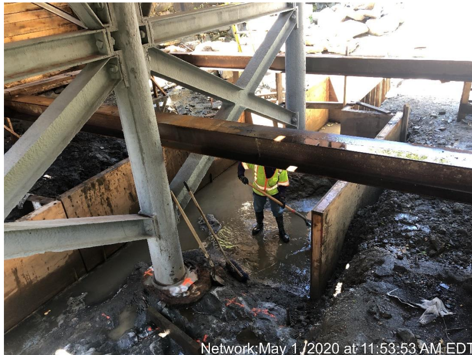
Cleaning the Pier Footing Formwork
