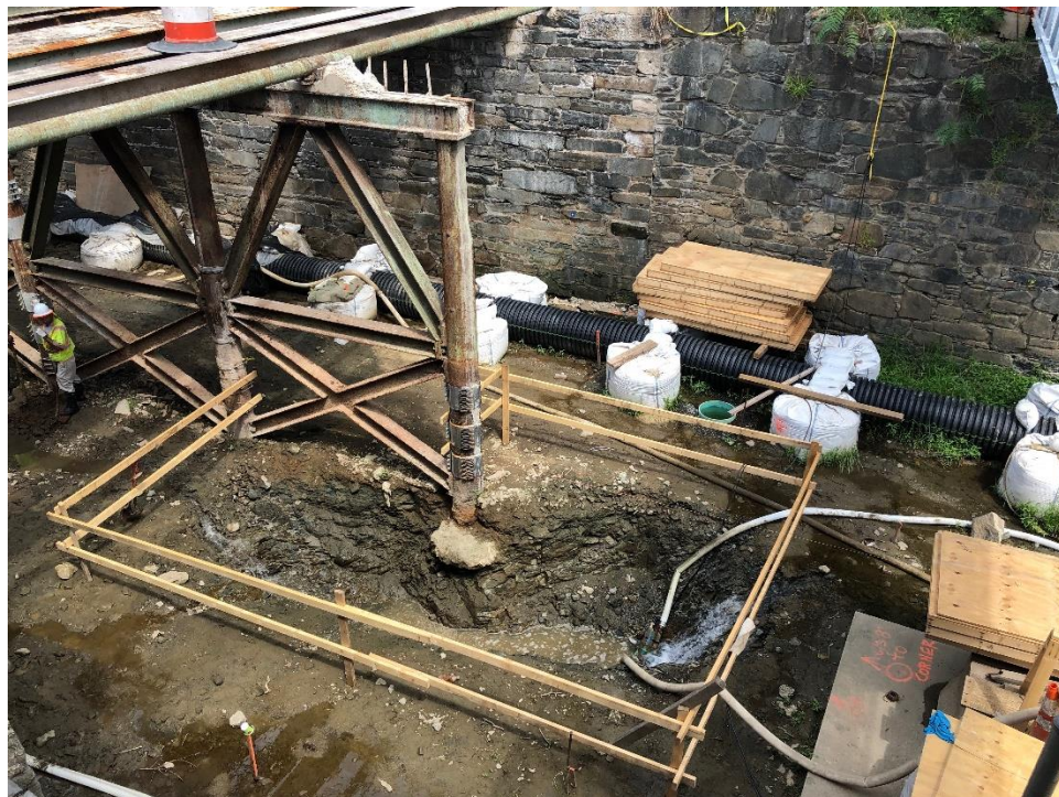
Dewatering the Work Zone
