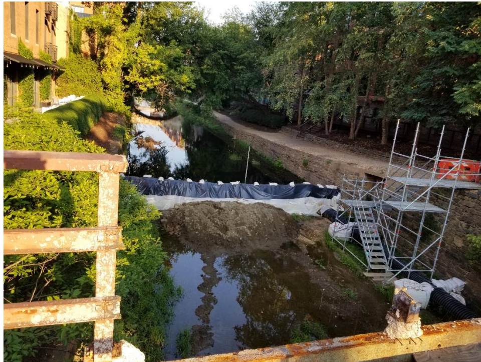
Downstream Side of the Western Cofferdam
