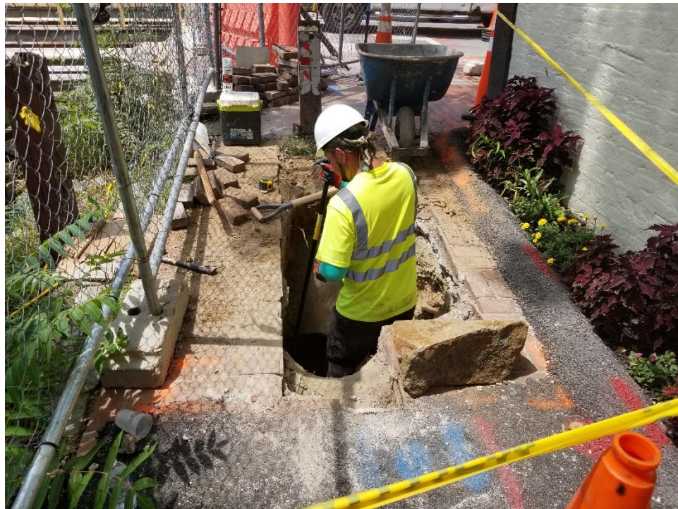
Test Pit for Water Main at the Northeast Side of the Bridge
