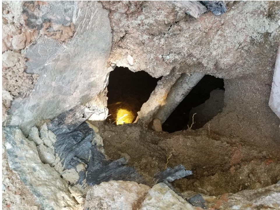
Void Encountered Under the Sidewalk
