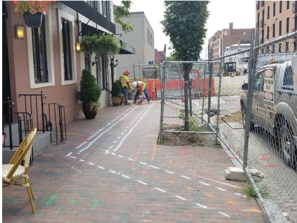
Saw Cut Demarcation for Water Main Relocation
