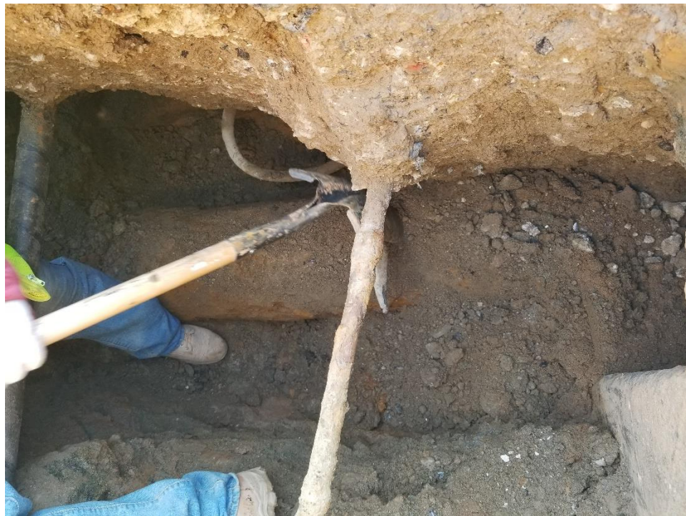
Locating Existing Water Main and Service Line North of the Bridge
