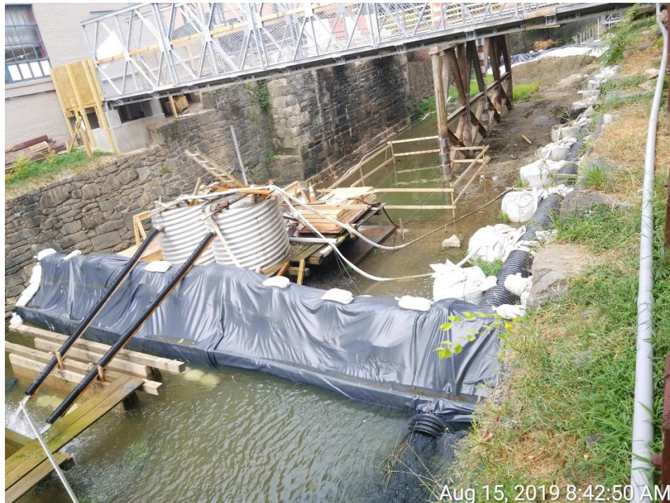
Work Zone Dewatering – East Side of the Canal
