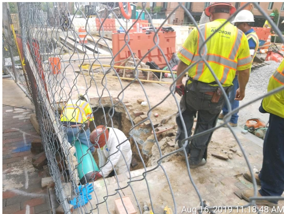
Replacing the Damaged Section of the Connect Pipe
