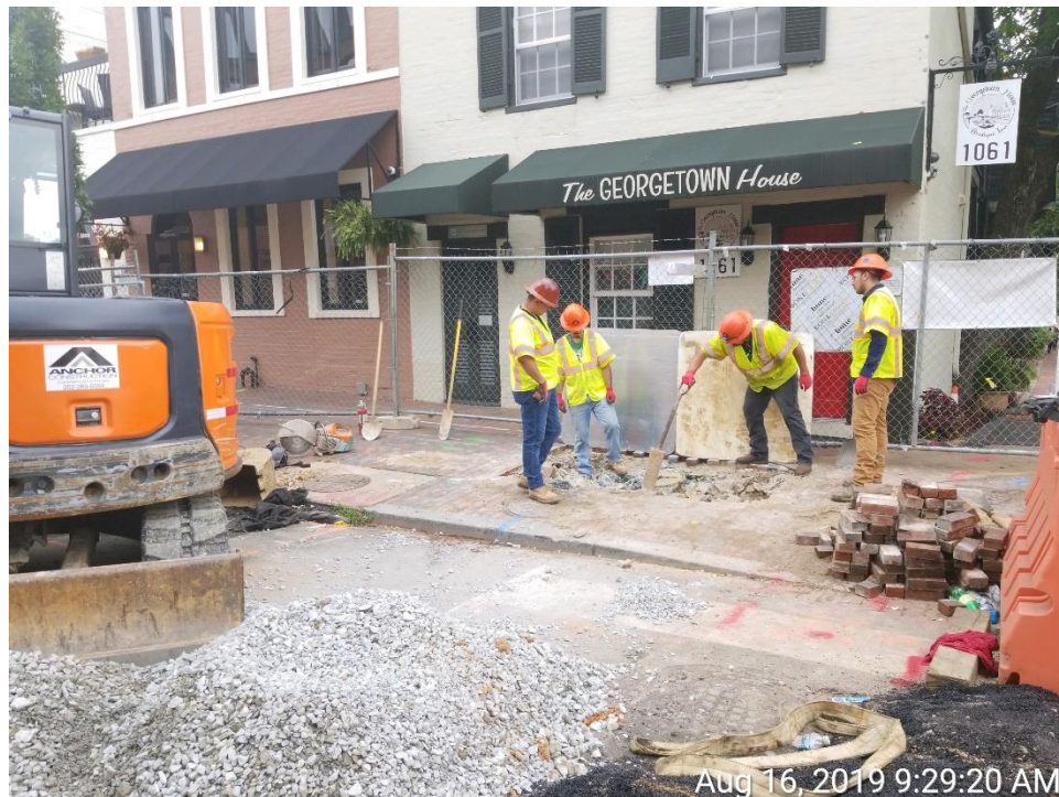
Repair Work of Existing Water Line - North Side of the Bridge
