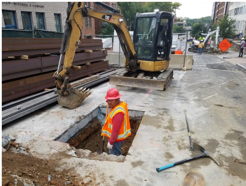
Test Pit for existing Water Main South of the Bridge
