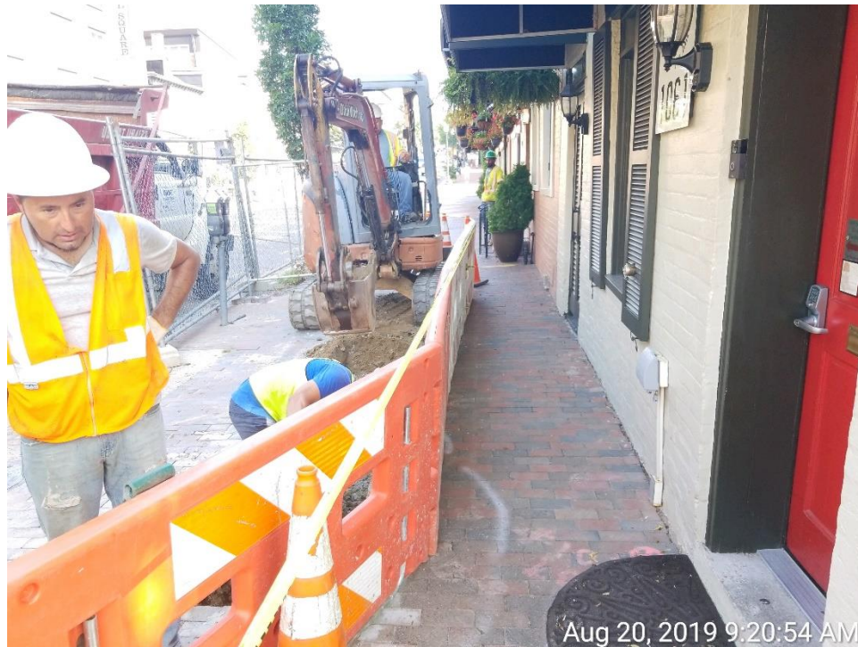
Maintaining the Sidewalk During Excavation for Water Main
