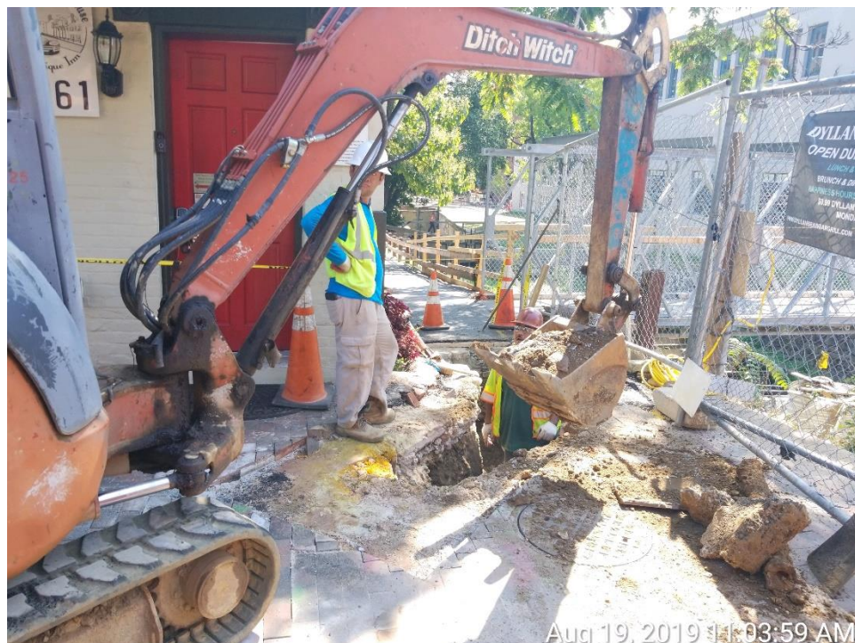
Water Main Relocation – Northeast Side of the Bridge
