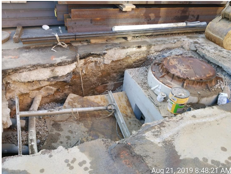
Installation of the New MCI Manhole South of Bridge
