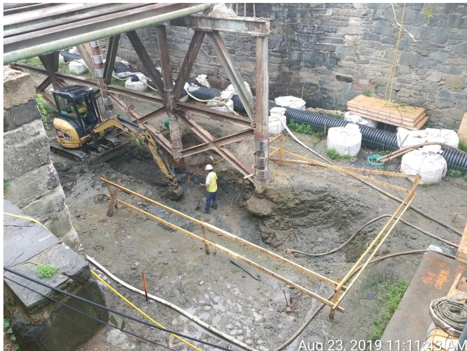
Excavation for the Pier Footings
