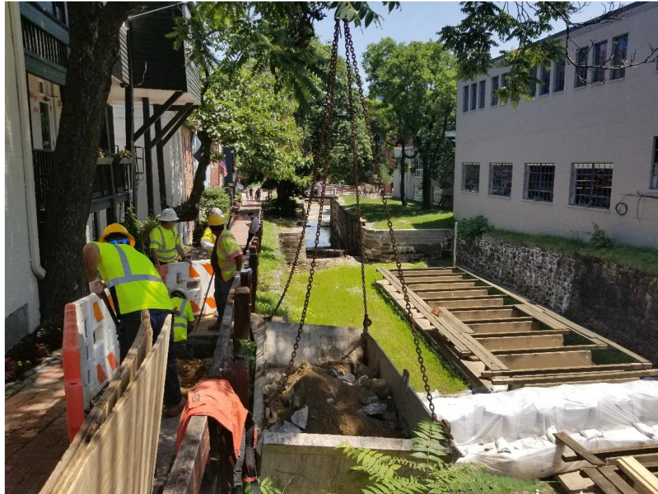
Excavation at the Temporary Pedestrian Bridge North Footing
