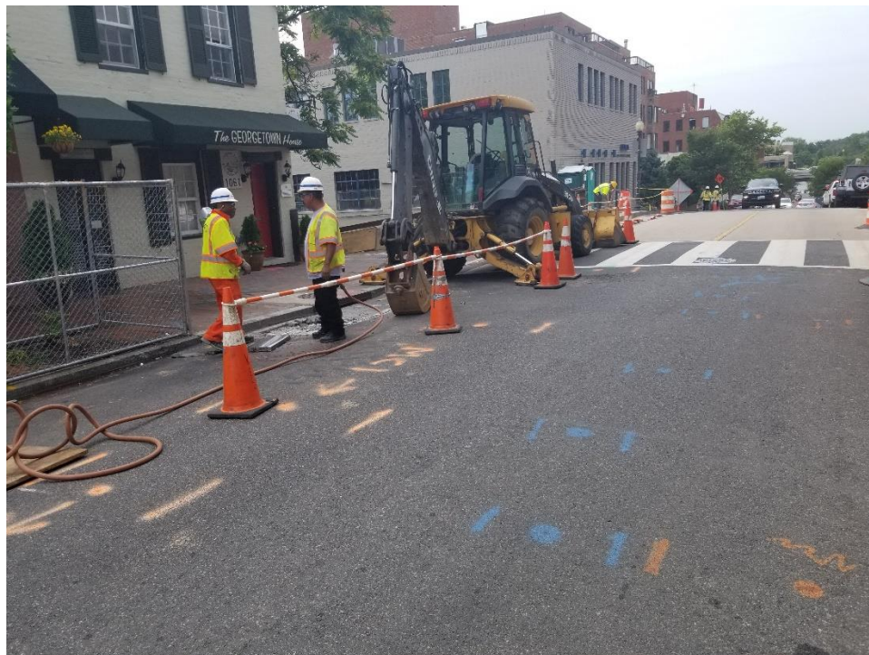
Washington Gas Conducting Cut/Tap of Existing Line on 31 st Street
