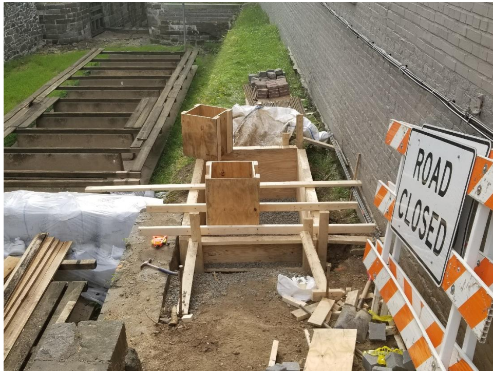
Installation of Formwork for the Temporary Pedestrian Bridge South Footing
