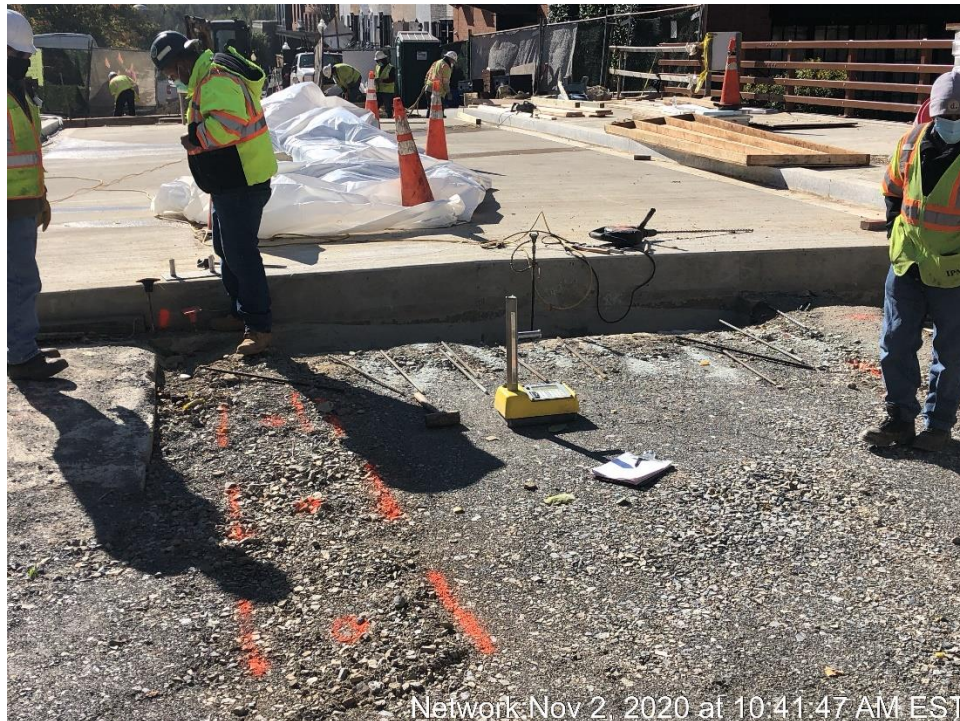
Density Testing for Aggregate Placed for Approach Slabs
