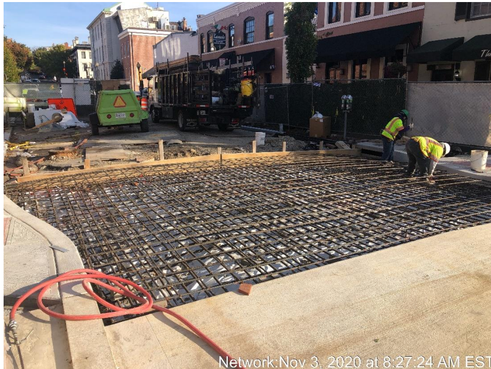
Reinforcing Steel for the Approach Slab North Side of the Bridge
