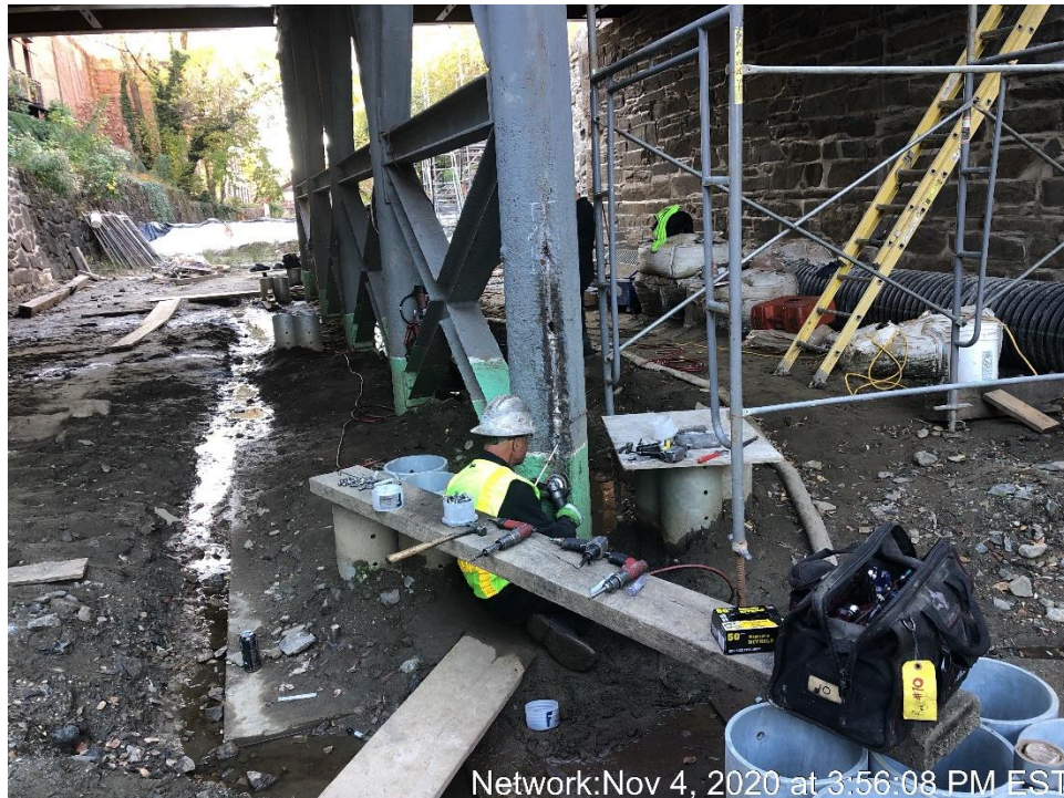
Lock and Stitch Repairs at Pier Column
