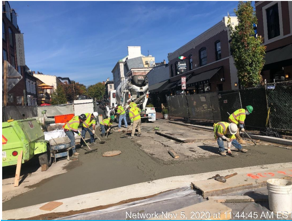
Placement of Concrete for PCC Pavement Repairs North Side of the Bridge
