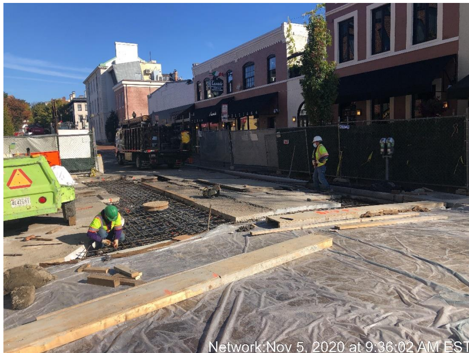
Reinforcing Steel for PCC Pavement Repairs North Side of the Bridge
