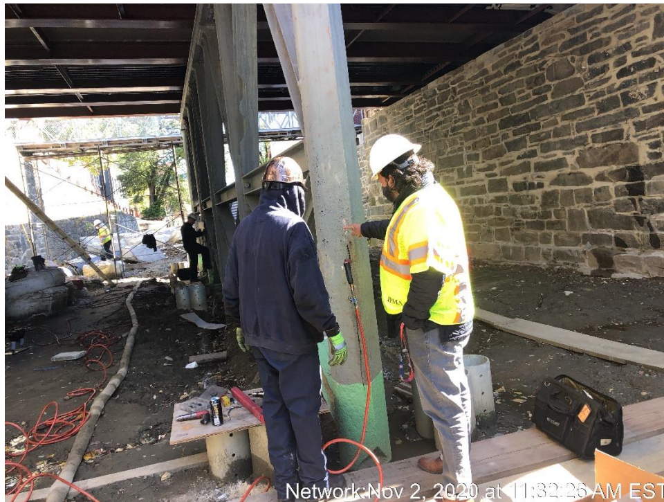
Lock and Stitch Repairs at Pier Column
