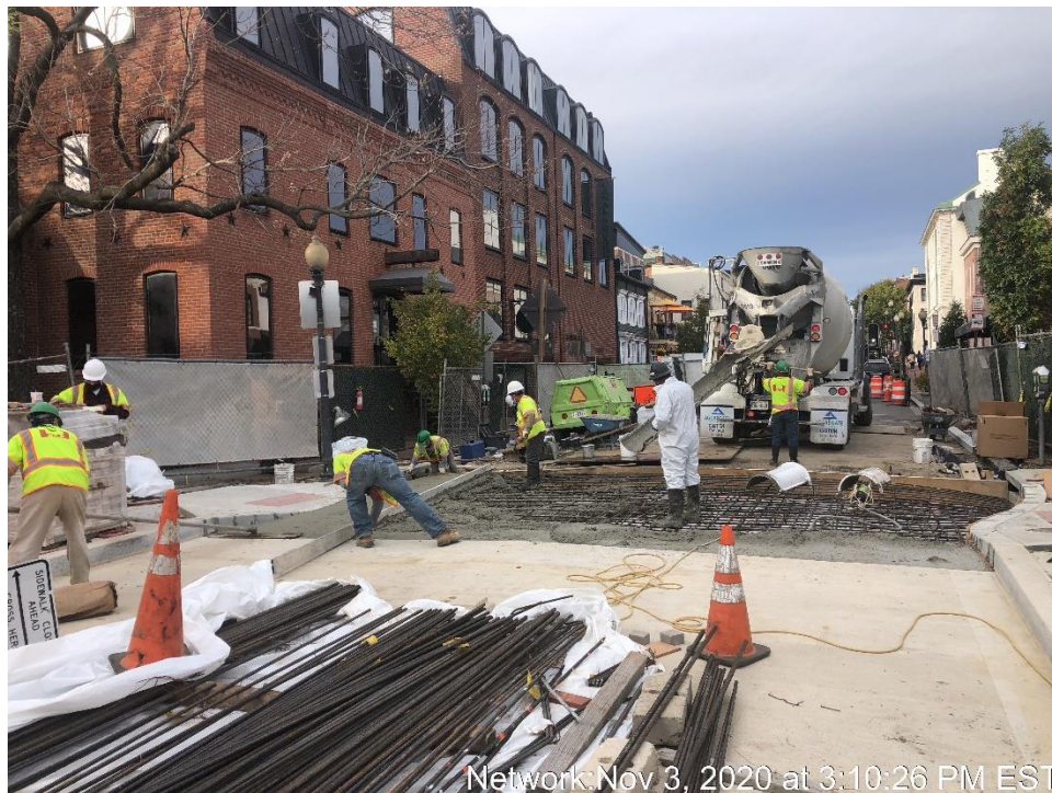
Placement of Concrete for Approach Slab North Side of the Bridge
