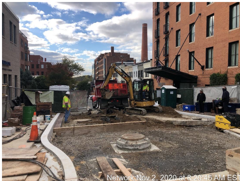
Excavation for PCC Pavement Repairs South Side of the Bridge
