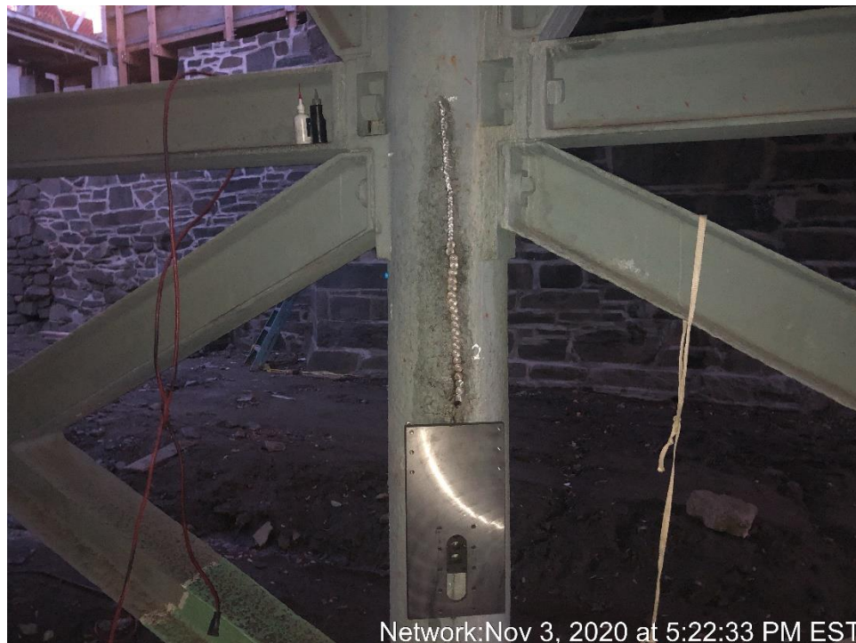
Lock and Stitch Repairs at Pier Column
