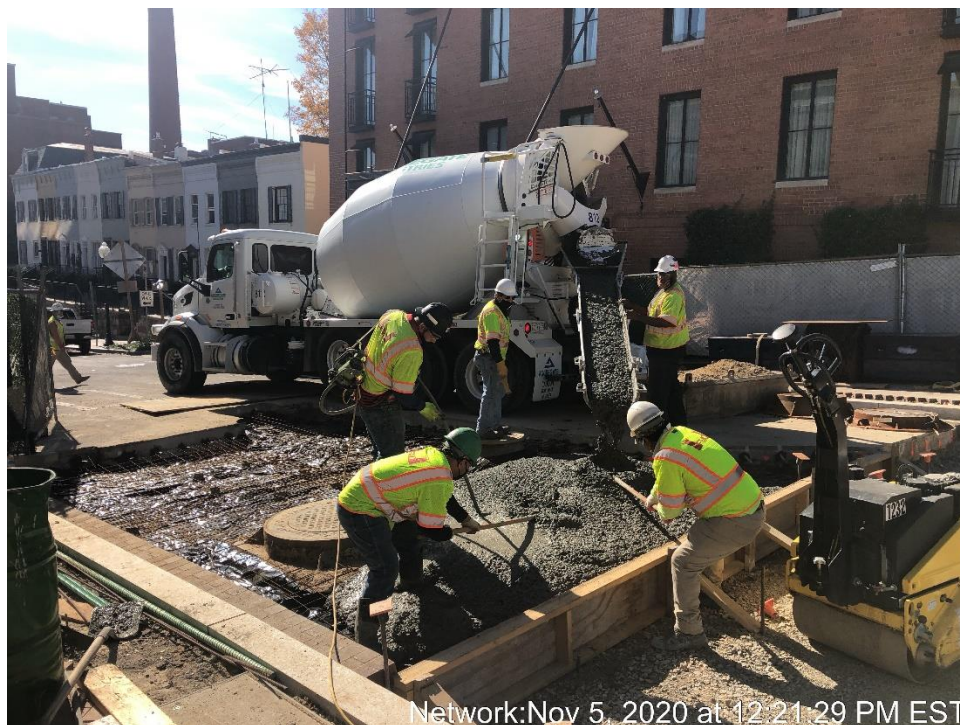
Placement of Concrete for PCC Pavement Repairs South Side of the Bridge
