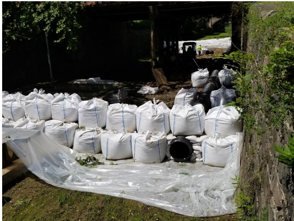
Installation of 24-inch Pipe
