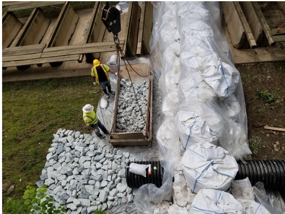
Placement of Rip Rap at the Pipe Outlet
