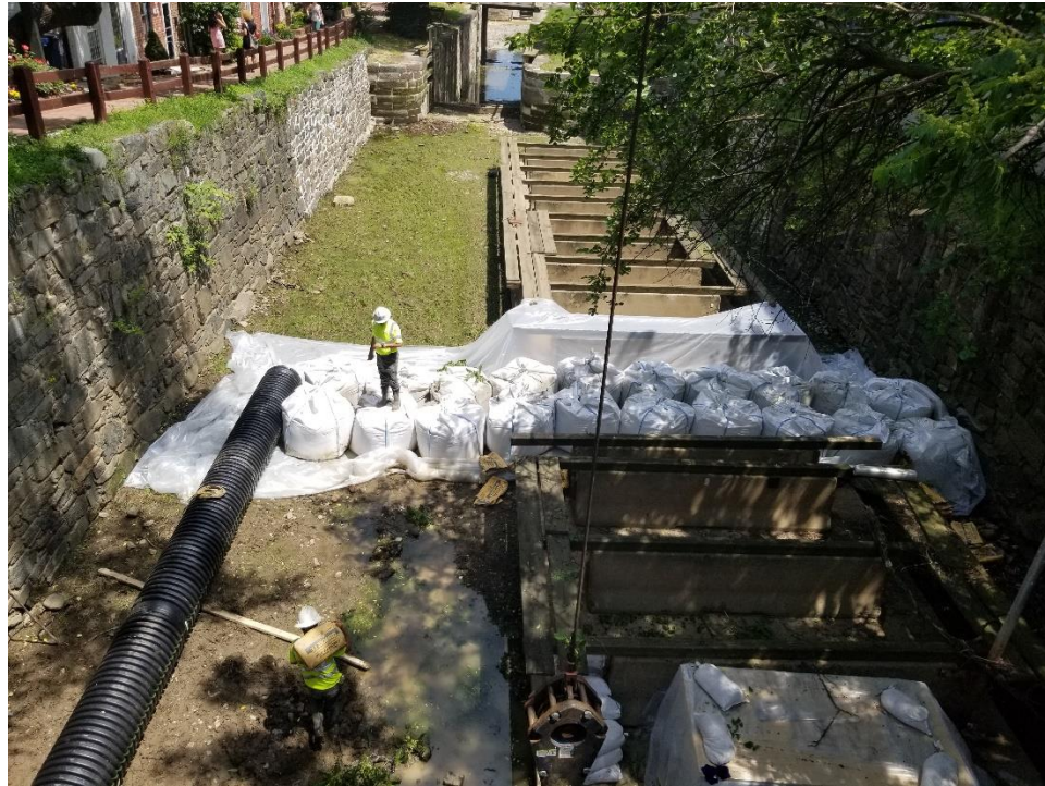
Cofferdam Construction East of the Bridge
