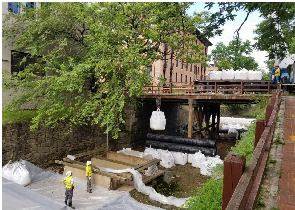
Cofferdam Construction East of the Bridge
