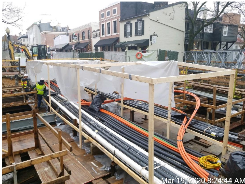
Removal of Asbestos Containment
