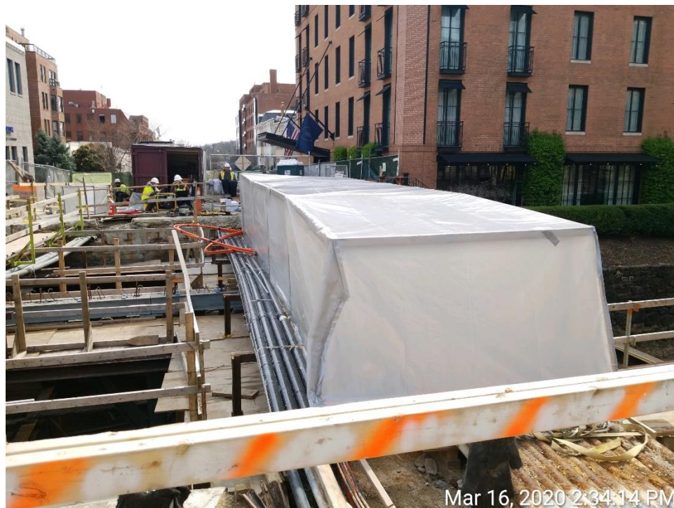
Verizon Installed the Asbestos Containment
