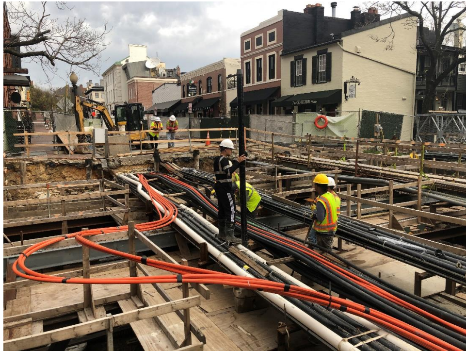
Installation of Split Duct - Verizon Cables
