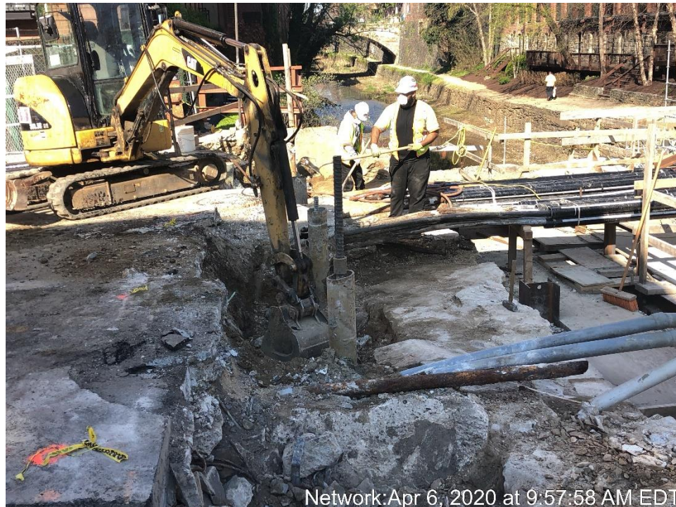
Back Wall Excavation and Stone Wall Removal at South Abutment
