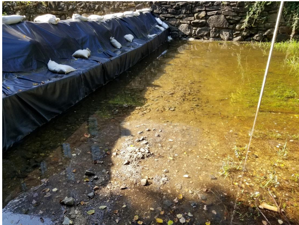
Canal Filling - Upstream Side of Cofferdam West of the Bridge
