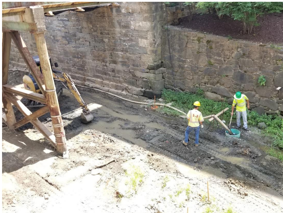
Water Pumping Station Inside the Work zone
