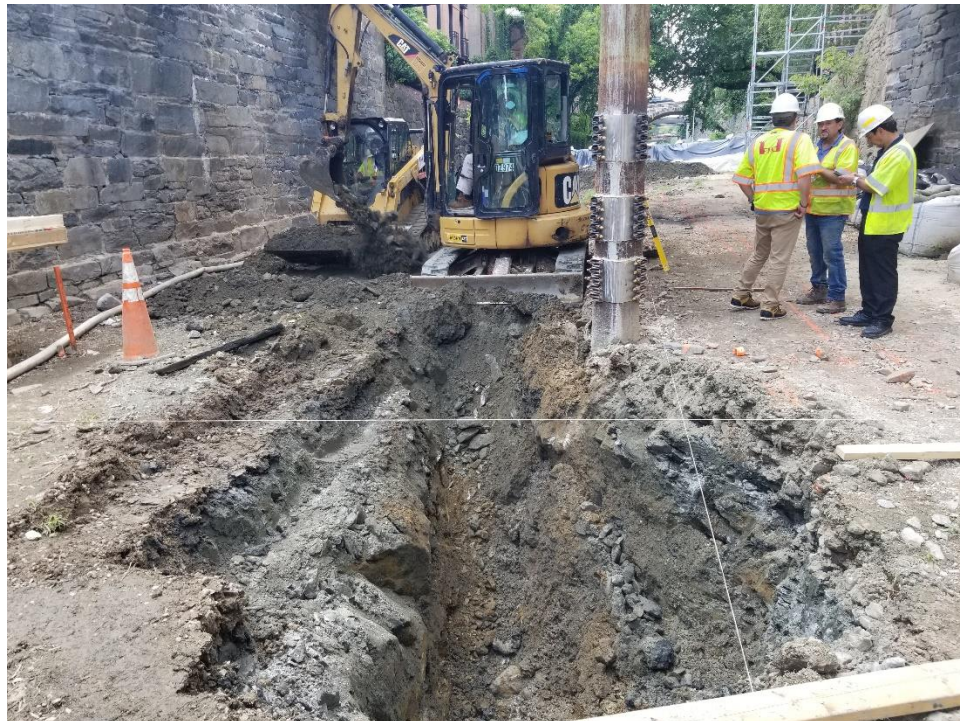
Excavation of Pier Footing – Pier #1
