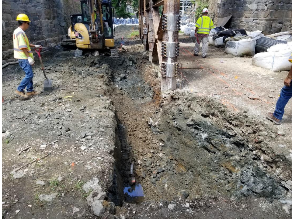
Excavation of Pier Footing – Pier #1
