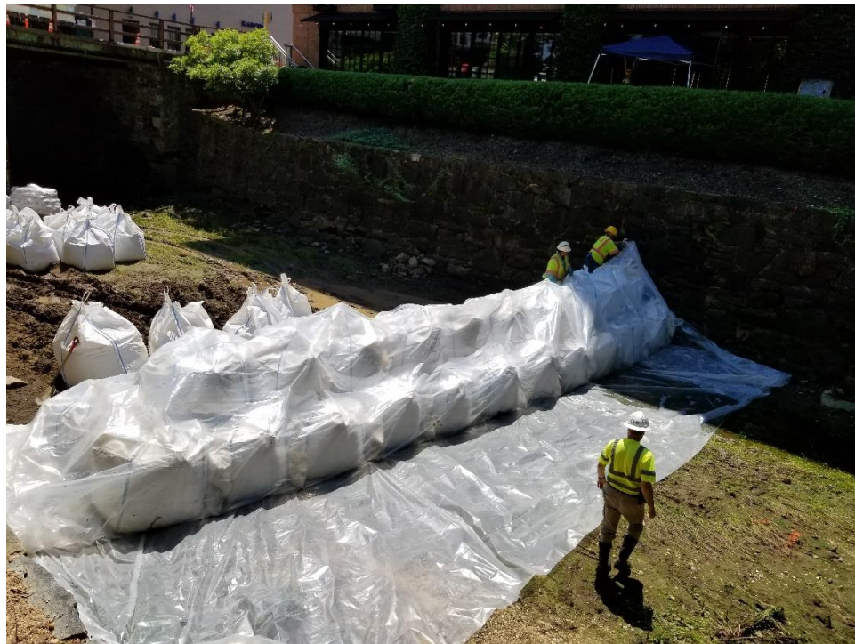
Construction of Cofferd Dam at the West Side of the Bridge
