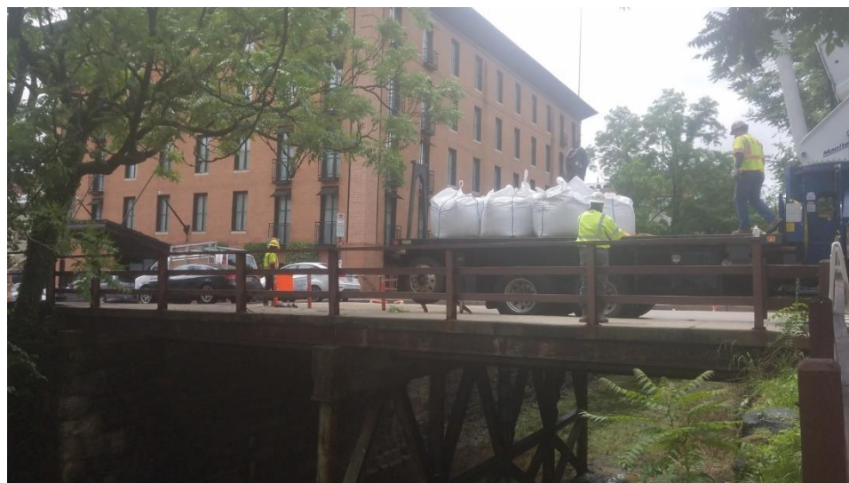
Delivery of Sand Bags
