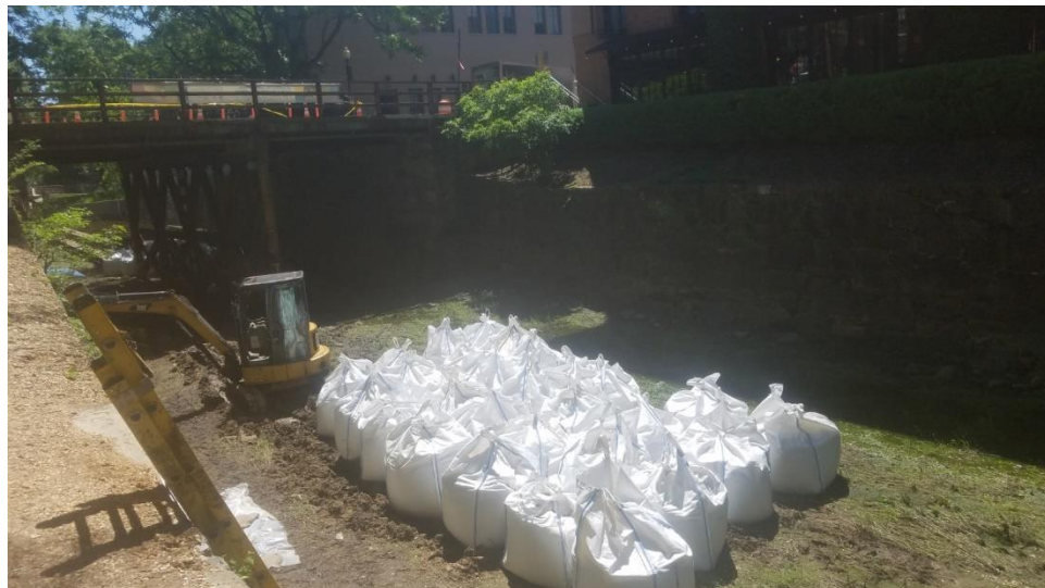
Sand Bags on the West Side of the Bridge
