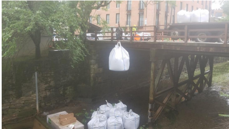
Lowering Sand Bags on East Side of the Bridge
