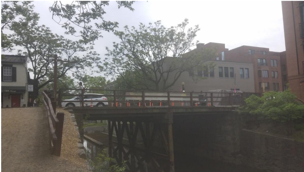
31 st Street Bridge over C&O Canal
