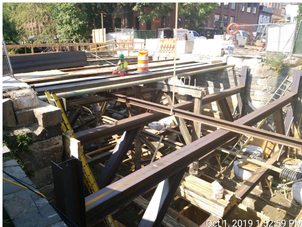
Installation of Canal Wall Support
