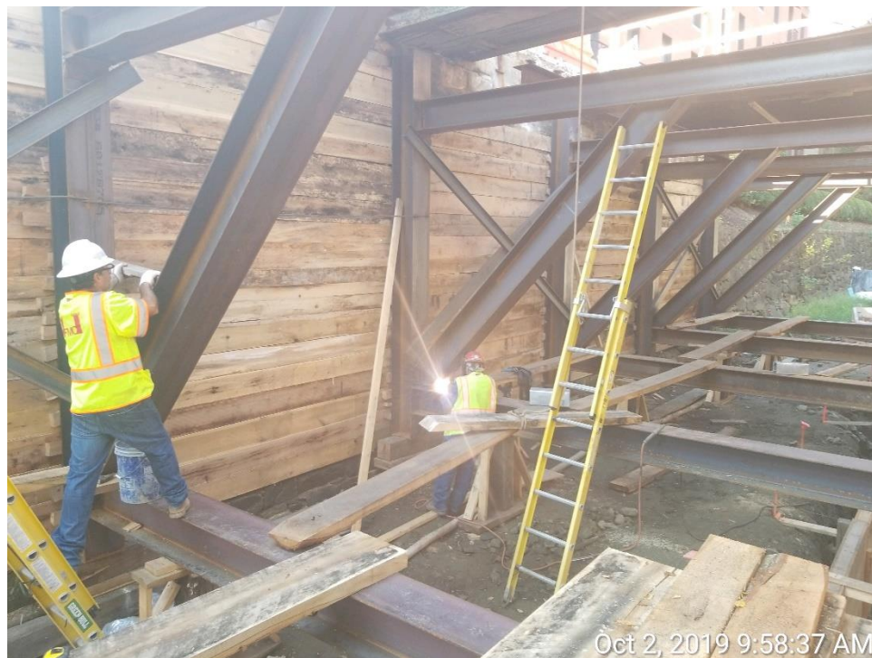
Installation of Canal Wall Support
