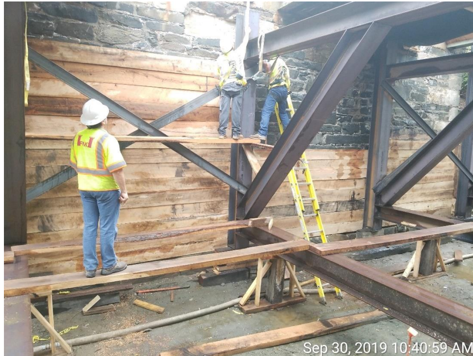
Installation of Canal Wall Support
