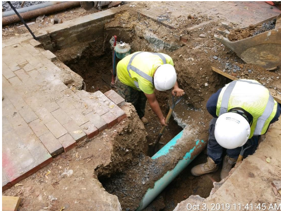
Preparation for Water Main Tie-in work
