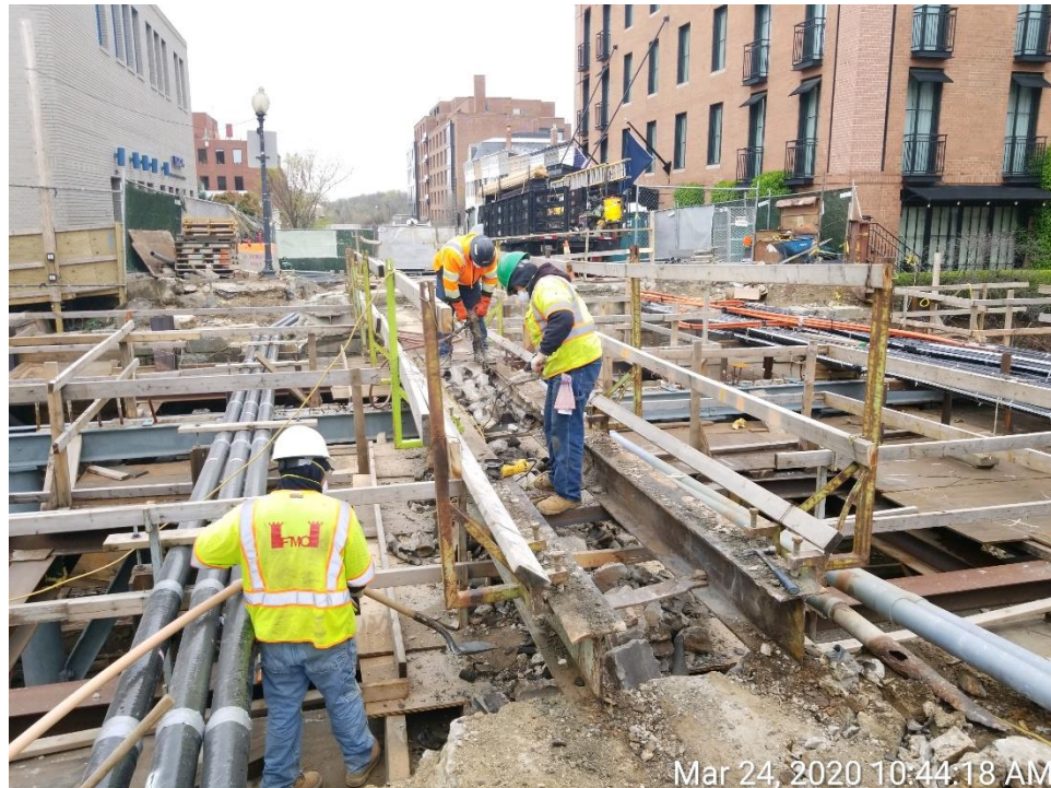
Demolition of Concrete Pepco Duct Bank
