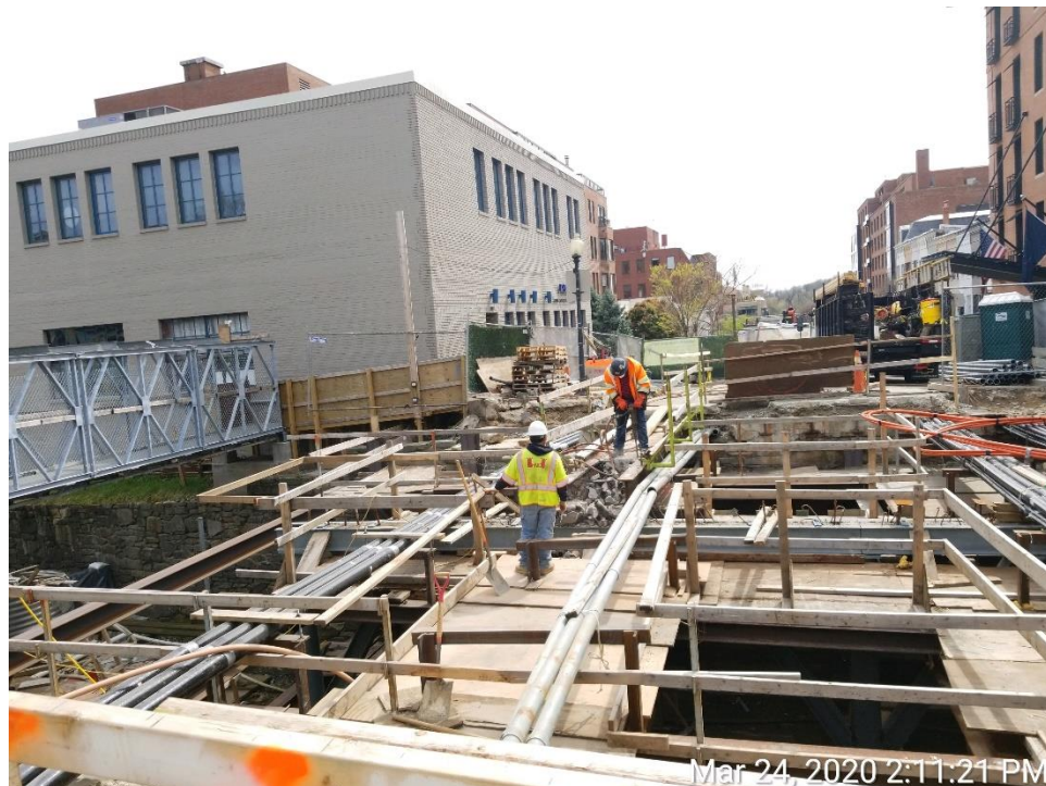
Demolition of Concrete Pepco Duct Bank
