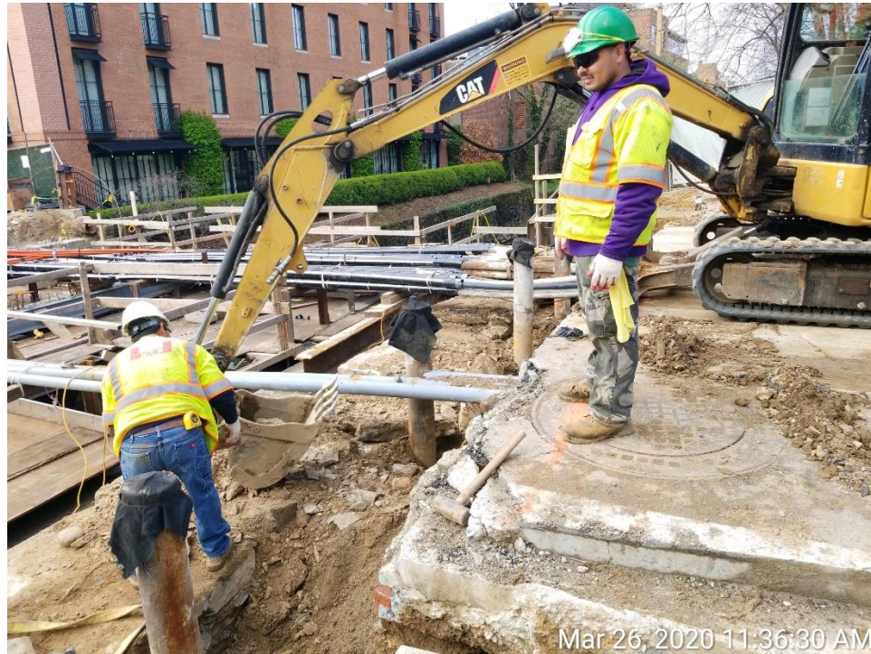
Back Wall Excavation at the North Abutment
