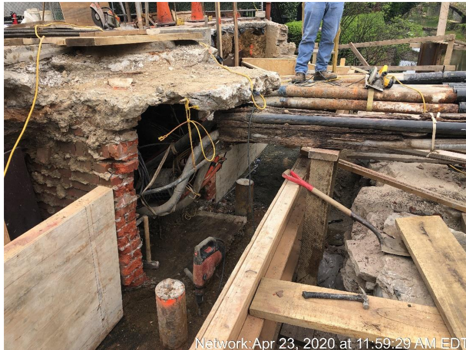
Excavation around Verizon Manhole – South abutment
