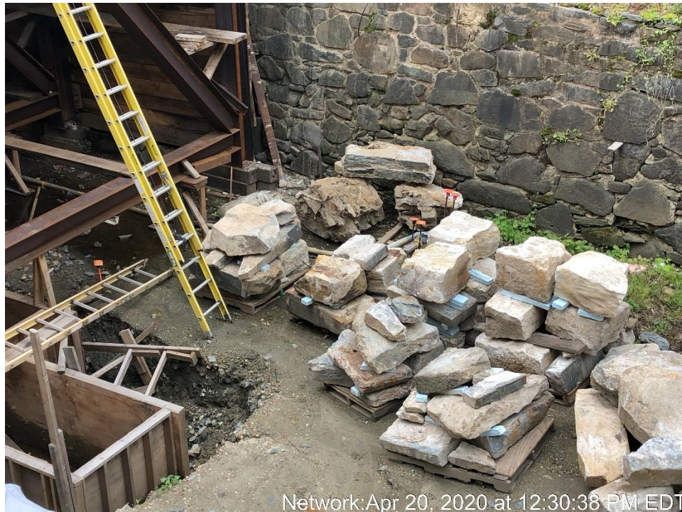
Storing Removed Canal Wall Stones Inside the Canal
