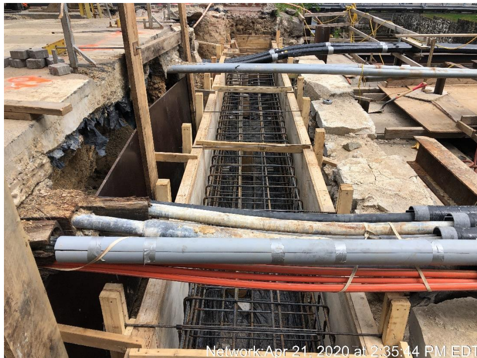
Placement of Reinforcing Steel at North Abutment Foundation
