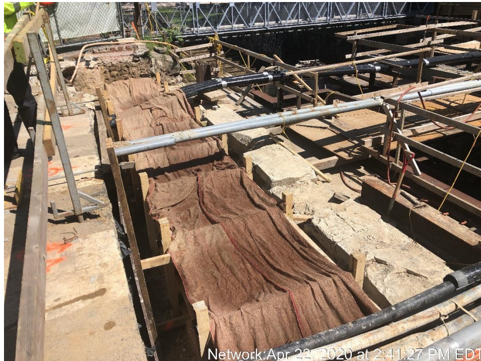
Concrete Curing – North Abutment Foundation
