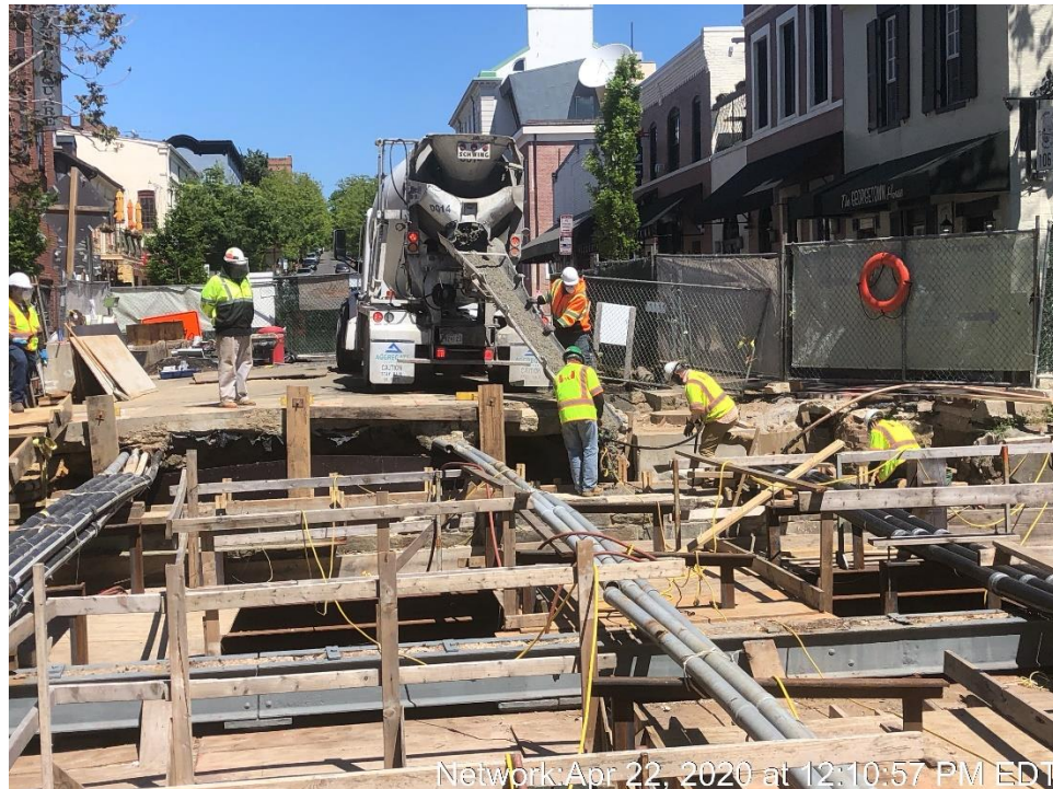
Placement of Concrete at North Abutment Foundation
