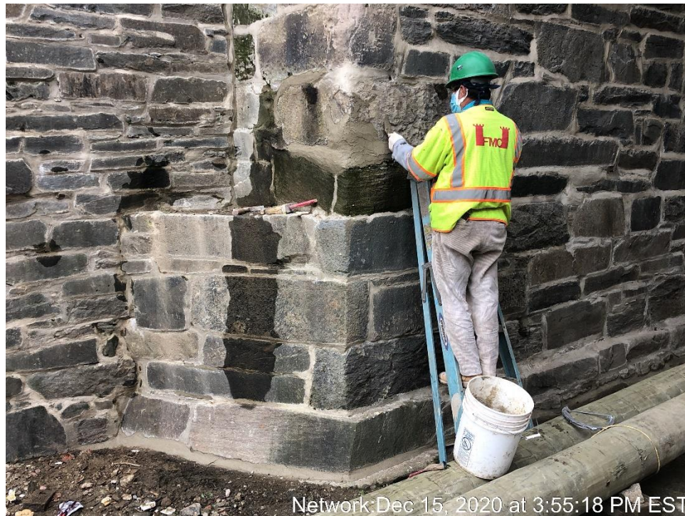
Repair and Repointing at the Canal's South Wall
