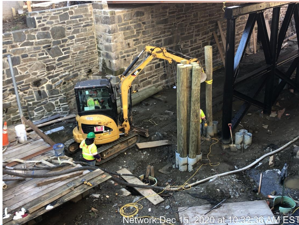
Installation of Timber Finder Around the Pier
