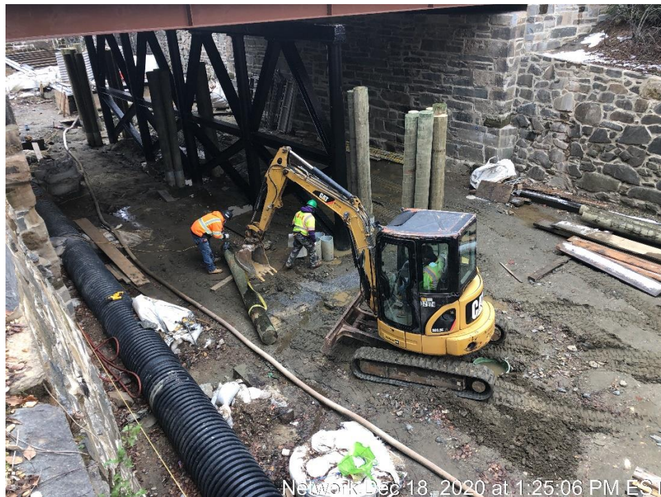
Installation of Timber Fender Around the Pier
