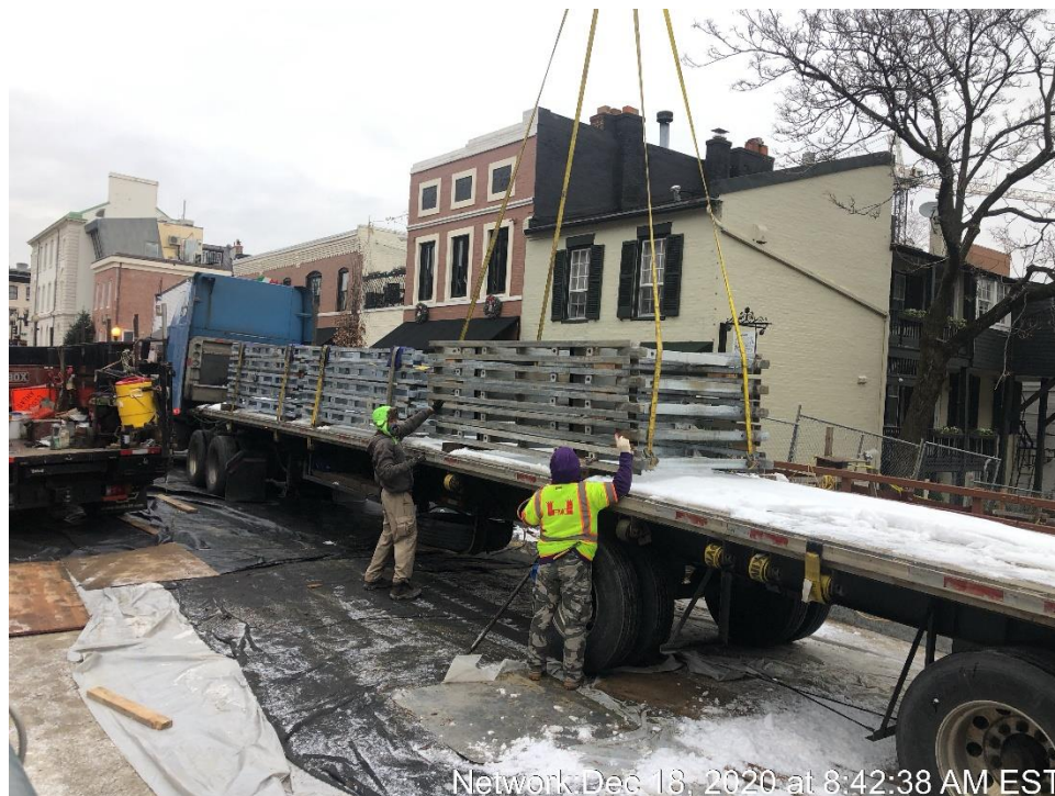
Removal of the Pedestrian Bridge from the Site
