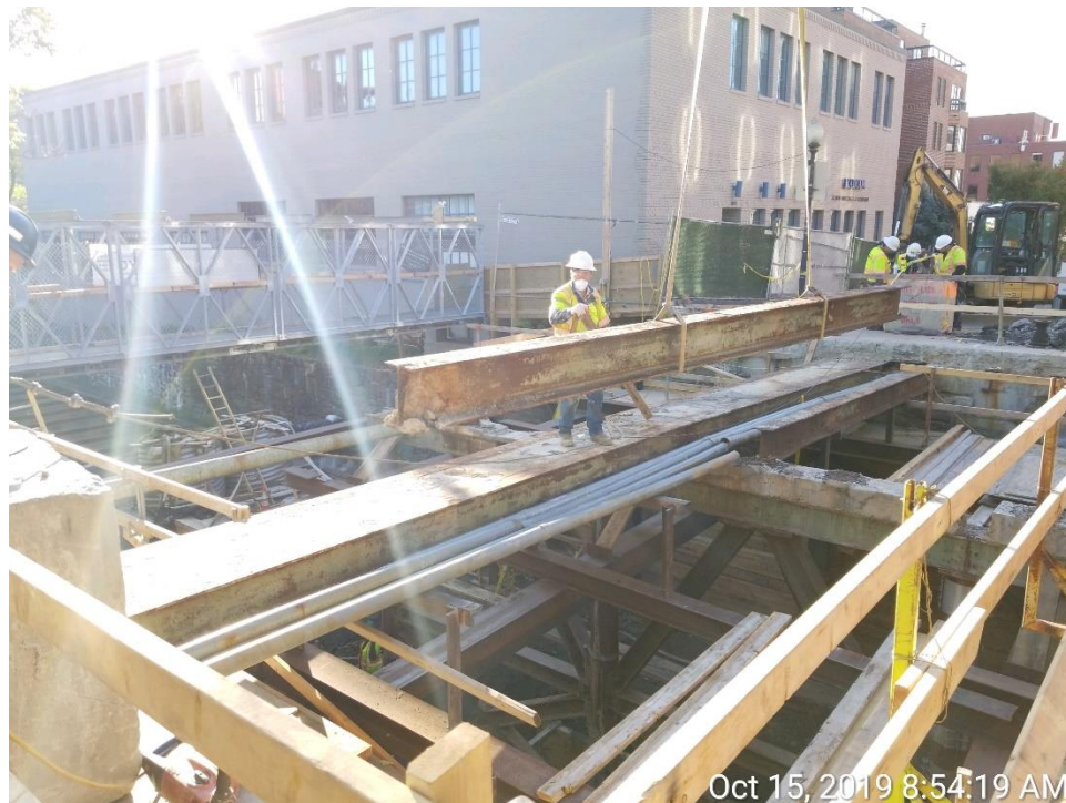
Demolition of Bridge Superstructure
