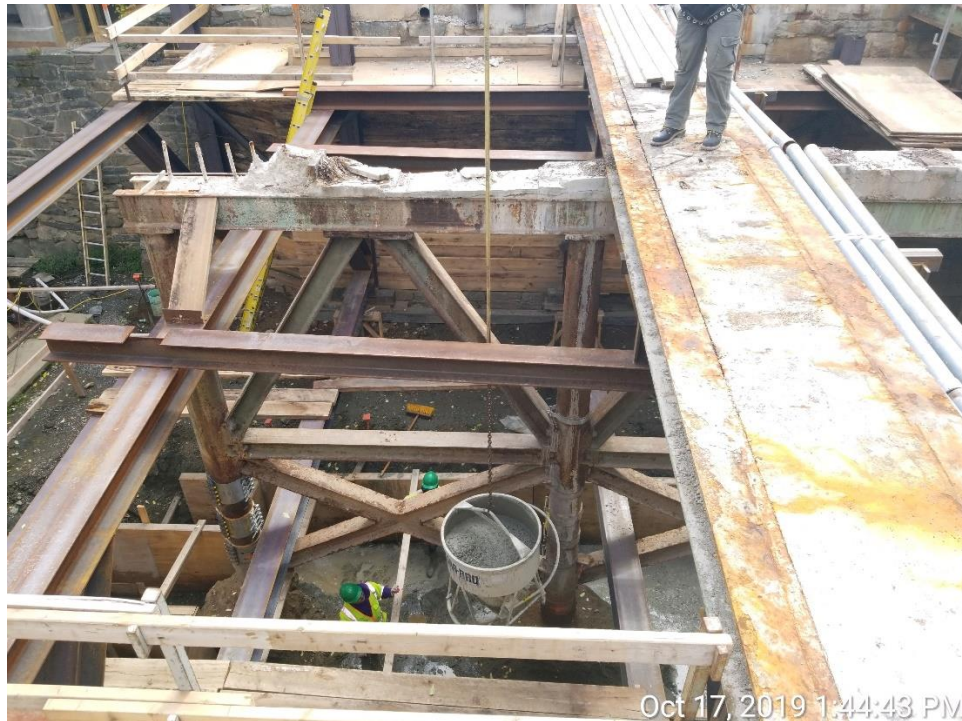
Concrete Placement for Mud Mat for Pier Foundation
