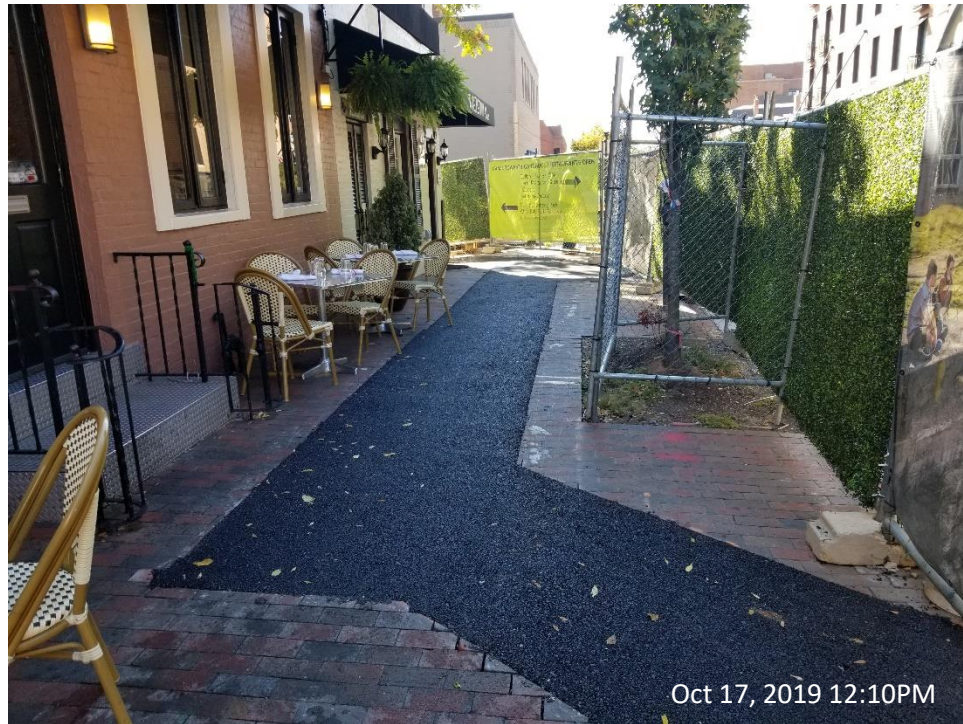
Placement of Asphalt for the Sidewalk in Front of Georgetown Inn
