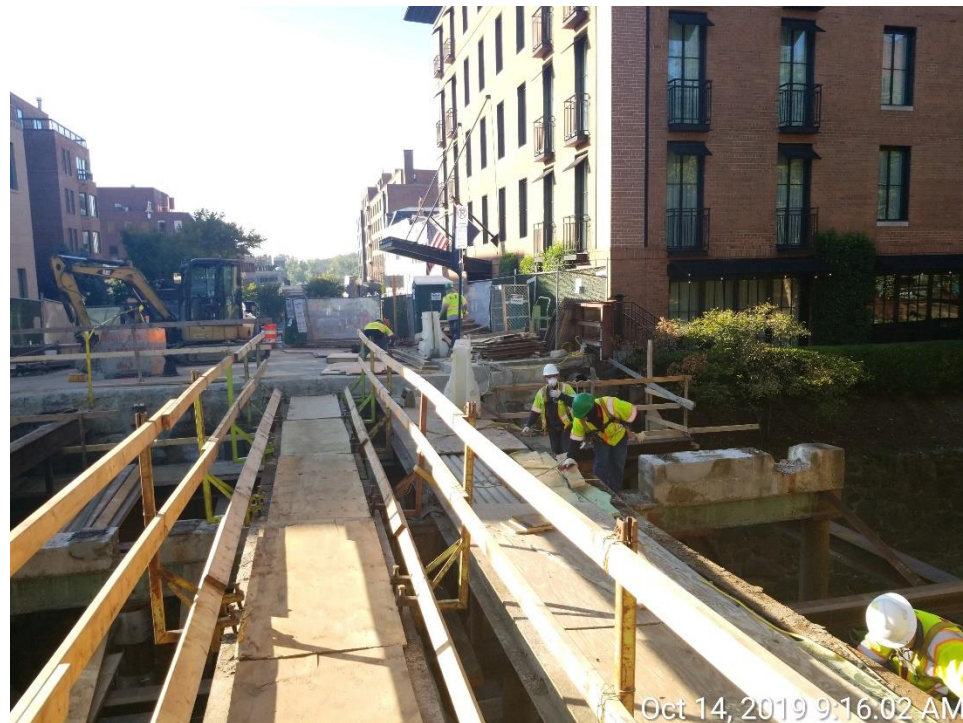
Demolition of Bridge Superstructure
