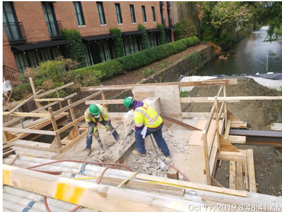
Demolition of Concrete Pier Cap on Top of Historic Pier
