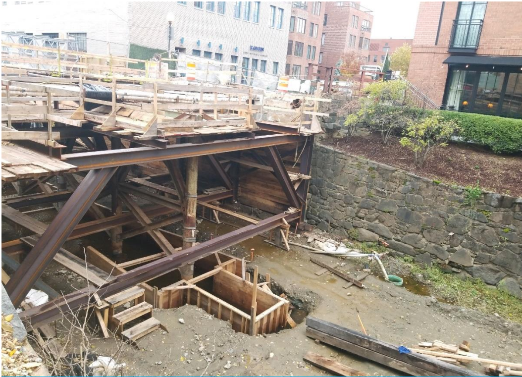
31 st Street Bridge over C&O Canal
