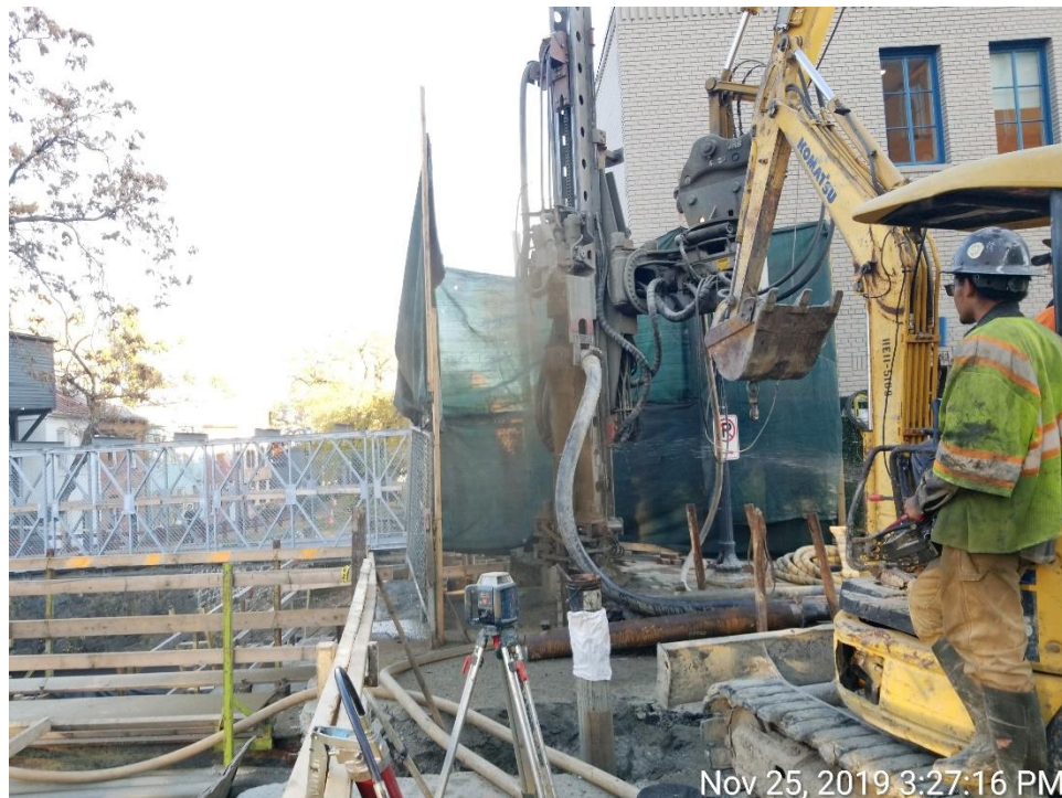
Drilling Pile #7
