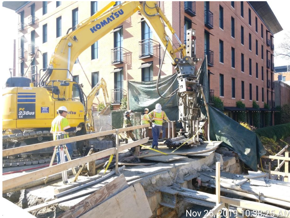
Drilling Pile #1
