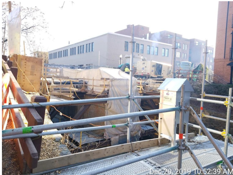
Containment for Pier Cleaning and Priming
