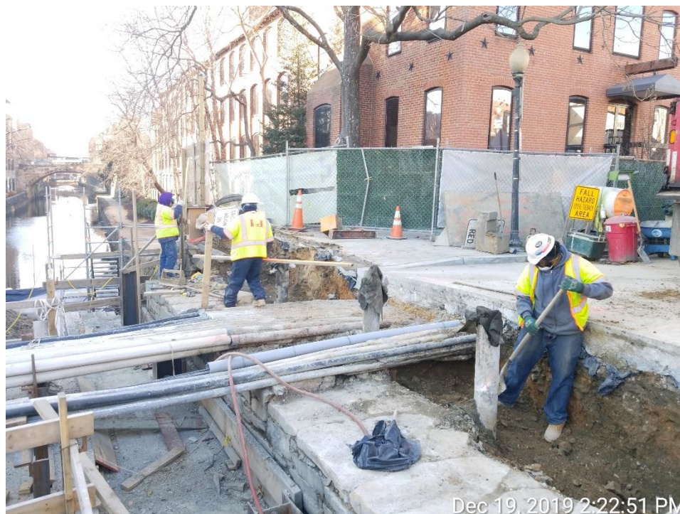
Excavation for the Bridge's North Abutment Footing
