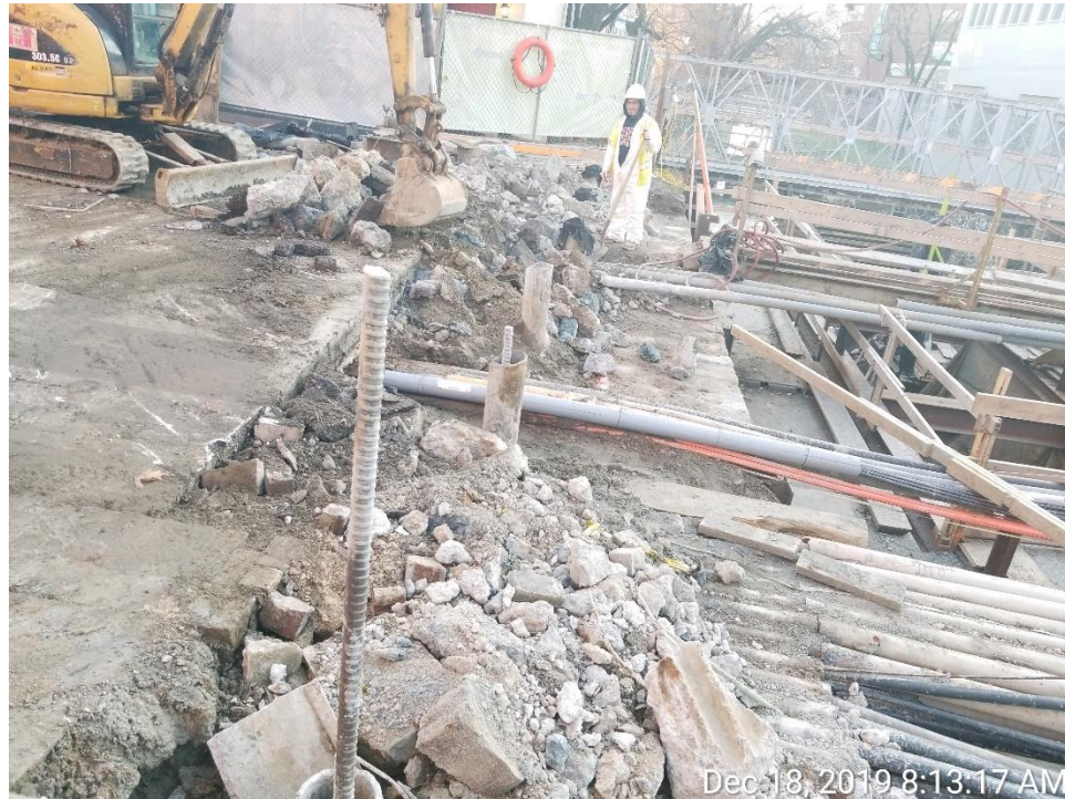
Excavation for the Footing at the North Side of the Bridge
