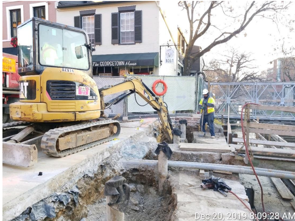
Excavation for the Bridge's North Abutment Footing
