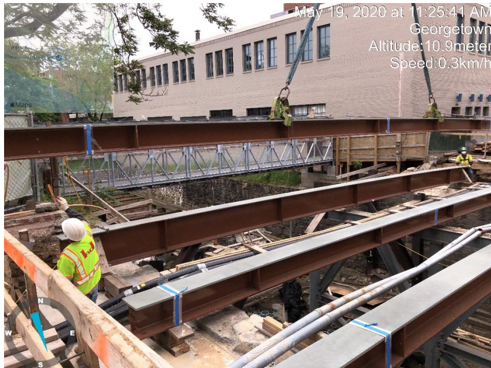
Delivery and Setting of Beams
