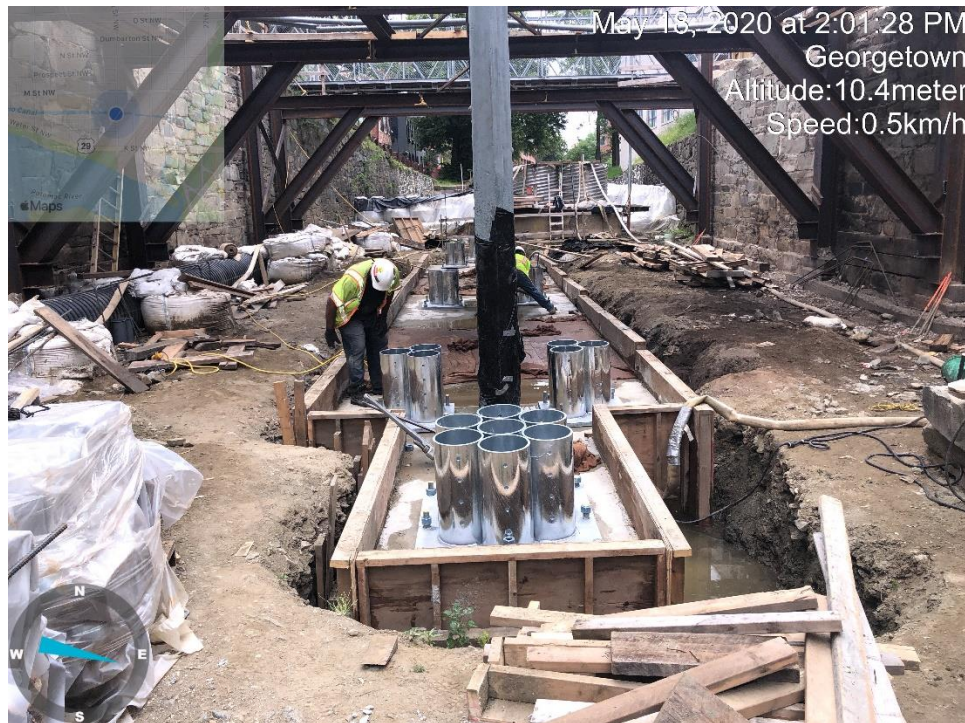
Installation of Dolphin Base Plate
