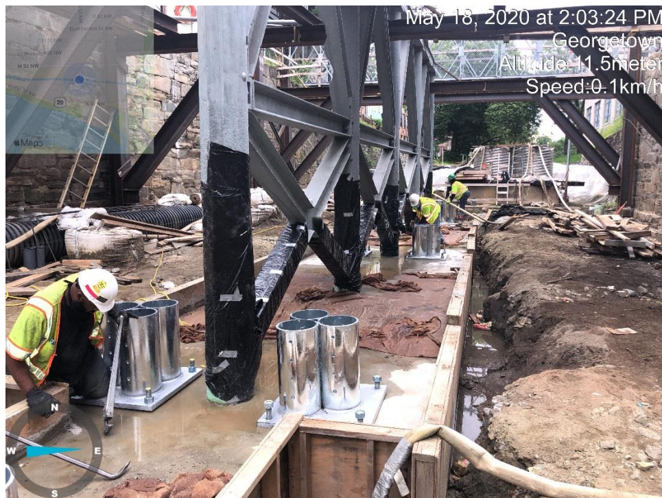
Installation of Dolphin Base Plate
