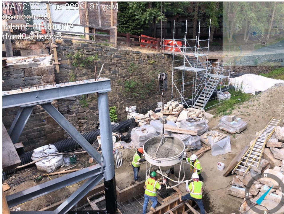
Placement of Concrete at Pier Footing
