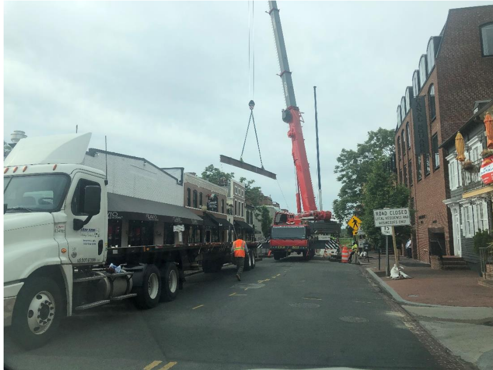
Delivery and Unloading of Beams
