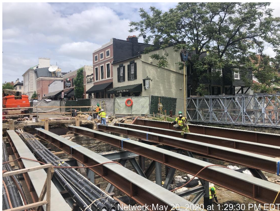
Setting of Beams
