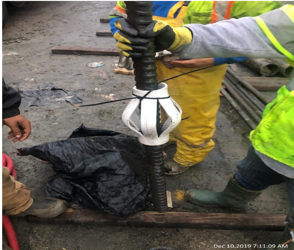
Placement of Reinforcement for Micropile – North Side of the Bridge
