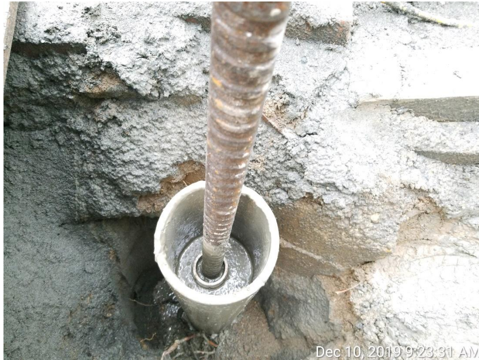
Micropile Grouting and Reinforcement – North Side of the Bridge
