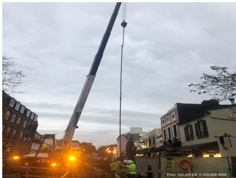
Placement of Reinforcement for Micropile – North Side of the Bridge
