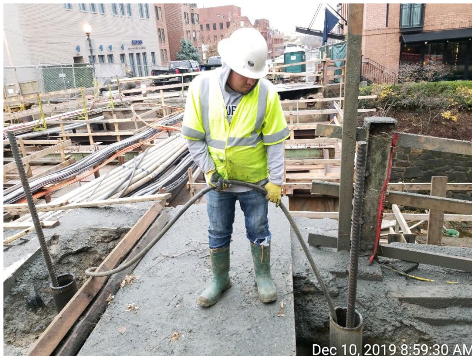
Micropile Grouting – North Side of the Bridge
