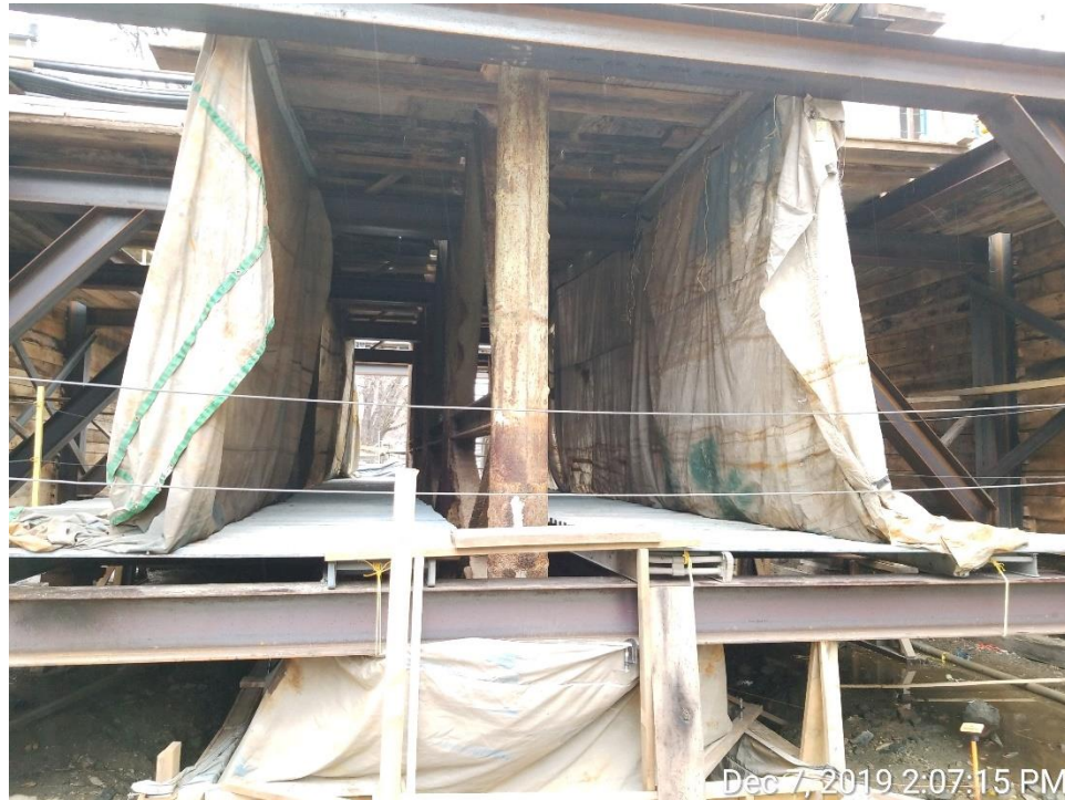
Cleaning and Painting Containment for the Historic Pier
