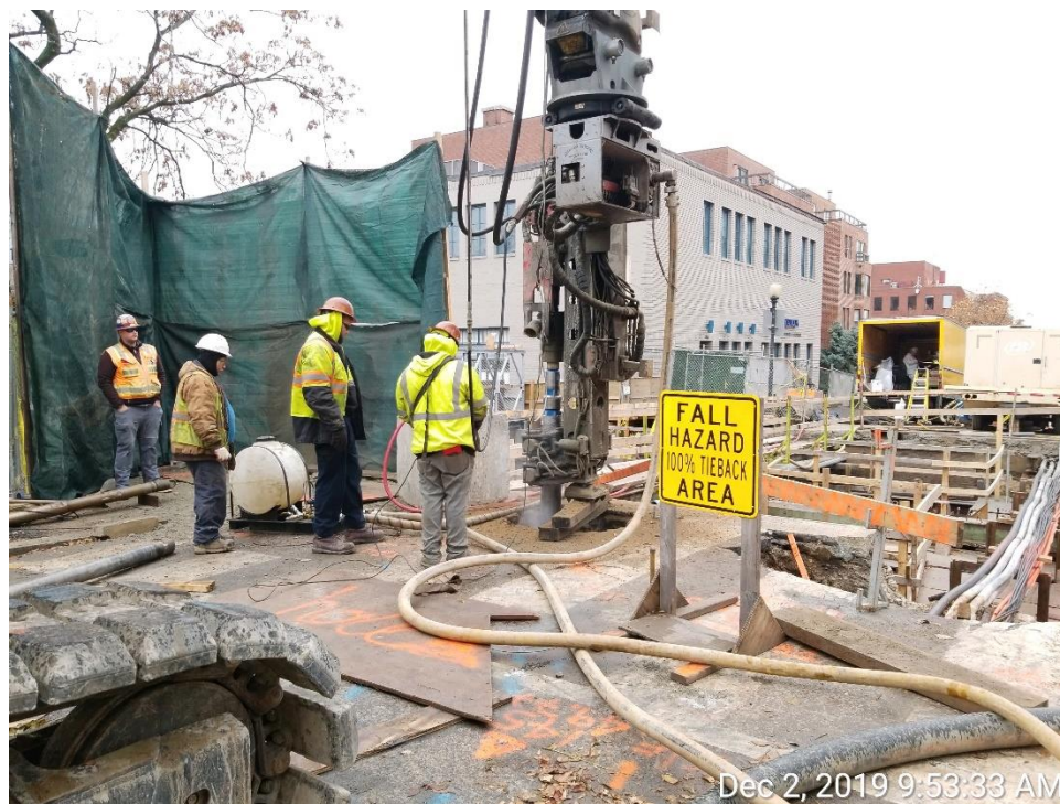
Micropile Drilling – North Side of the Bridge
