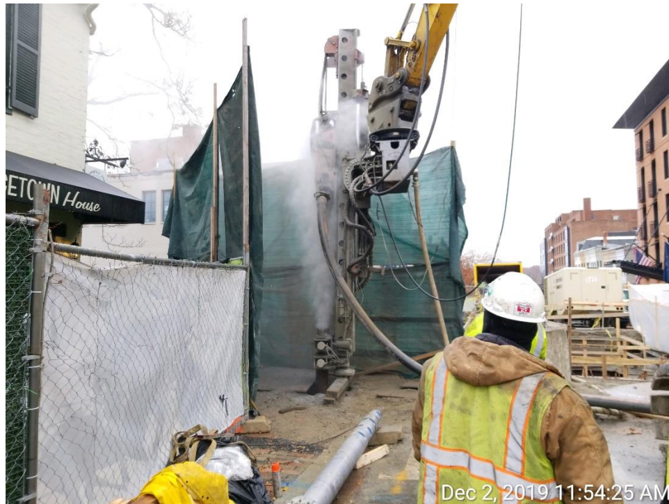
Micropile Drilling – North Side of the Bridge
