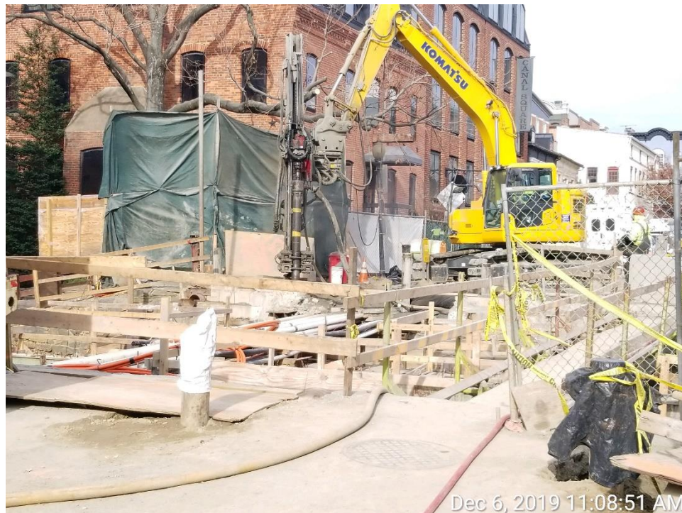
Micropile Drilling – North Side of the Bridge
