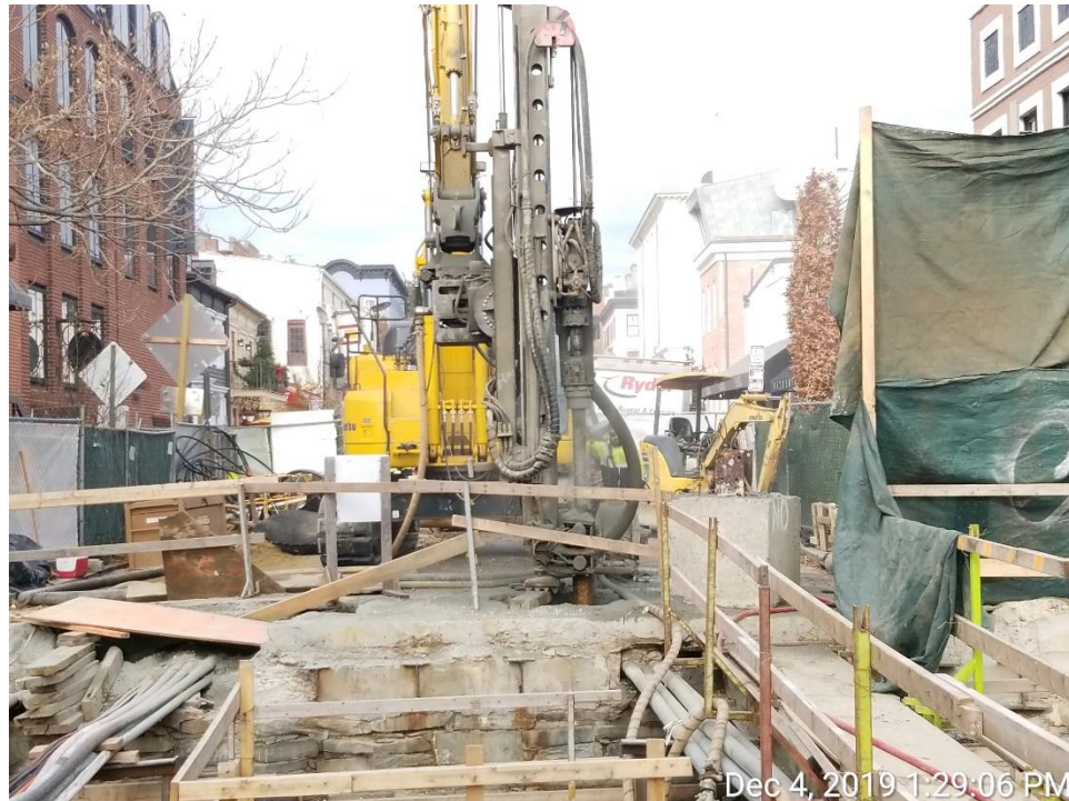
Micropile Drilling – North Side of the Bridge
